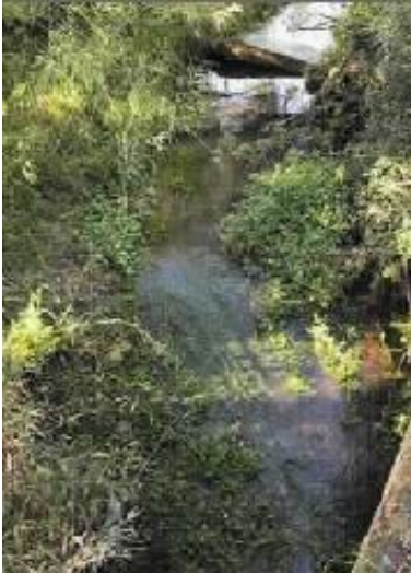
Figure 10 - Macroinvertebrate sample site on Mill River (56160)
