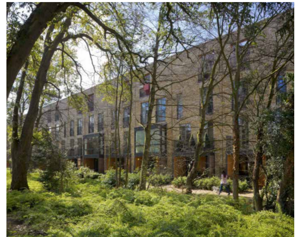
Accordia housing development, Cambridge UK
