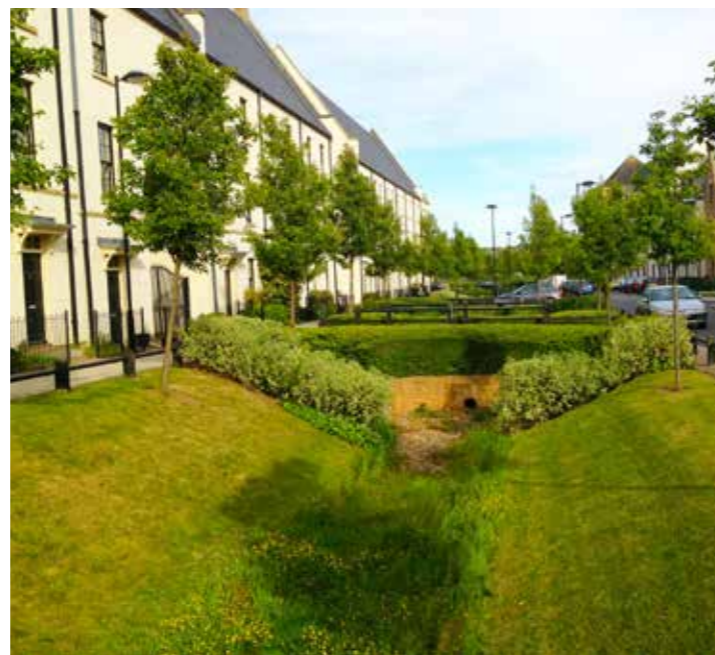
SuDS swale drainage and landscaping along the urban blocks
