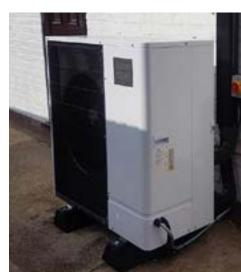
The fluid then passes through a compressor that raises it to a higher temperature, which can then heat water for the heating and hot water circuits of the house.
