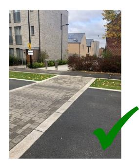
Fig 11 Swales is slabbed to allow 1100 litre bins to be easily moved to the roadside for collection
