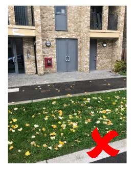
Fig 10 Swales mean there is no smooth access from bin store & bins have to be dragged across grass
