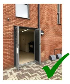
Fig 6 Double doors – stay open while collection takes place, with door bolts, hooks or automatic opening systems
