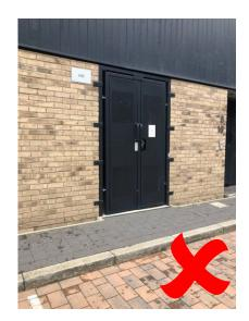
Fig 7 No drop kerb & pavement too narrow for 1100 litre bins
