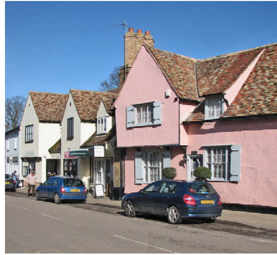
High Street Gables, Fulbourn
