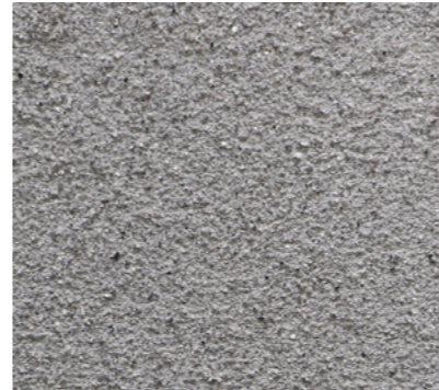
F4. Concrete Paving
