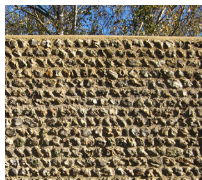
Feature Flint Wall
