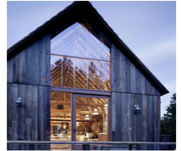
Local Timber Boarding
