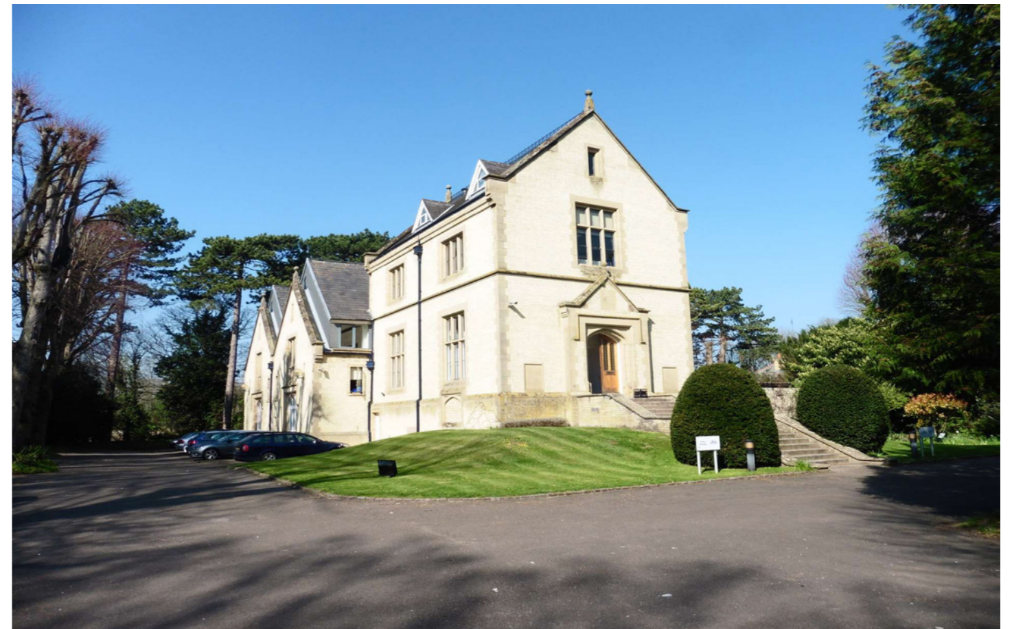
Figure 10. Pumping Station, Cow Lane
