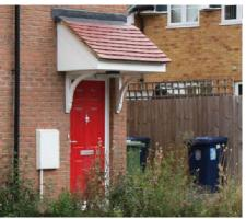
Fig. 73 - Prominent electric box and heavy porch details can spoil a facade
