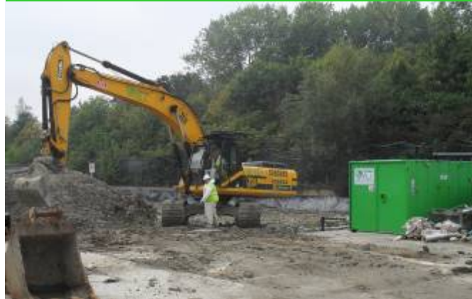
Constructing Ventilated Beds
