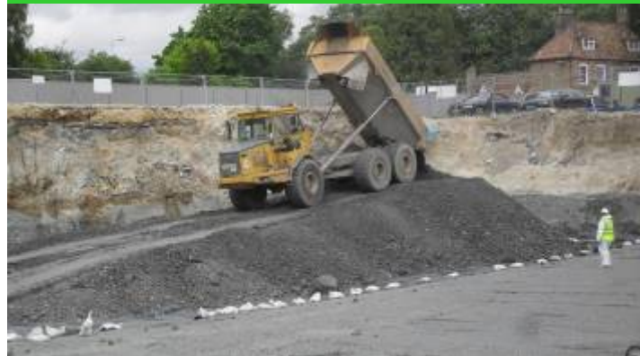
Stockpiling treated soils
