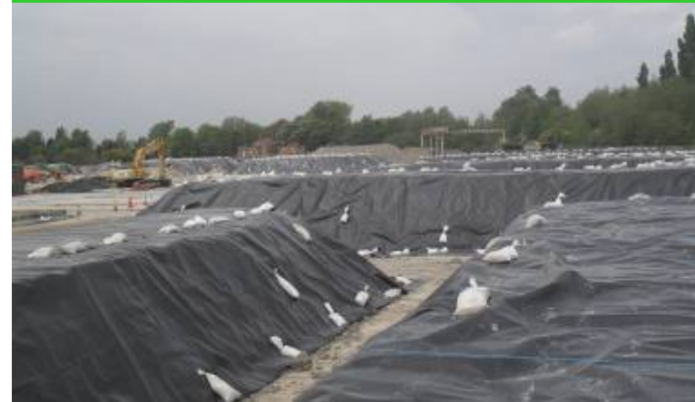
Covered Odourous Treatment Beds
