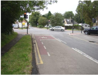
Advance stop lines are provided on the Regional Cycle network route at Oakington cross roads
