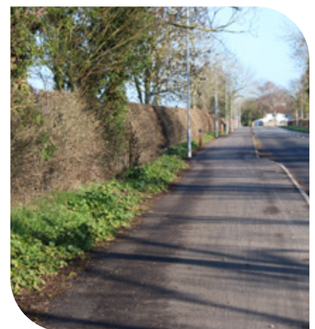
| New Road, Barton and the upgraded shared-use path, part of the Barton Greenway.
