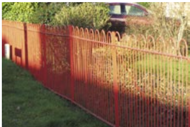
Hooped railings at No. 14 High Street
