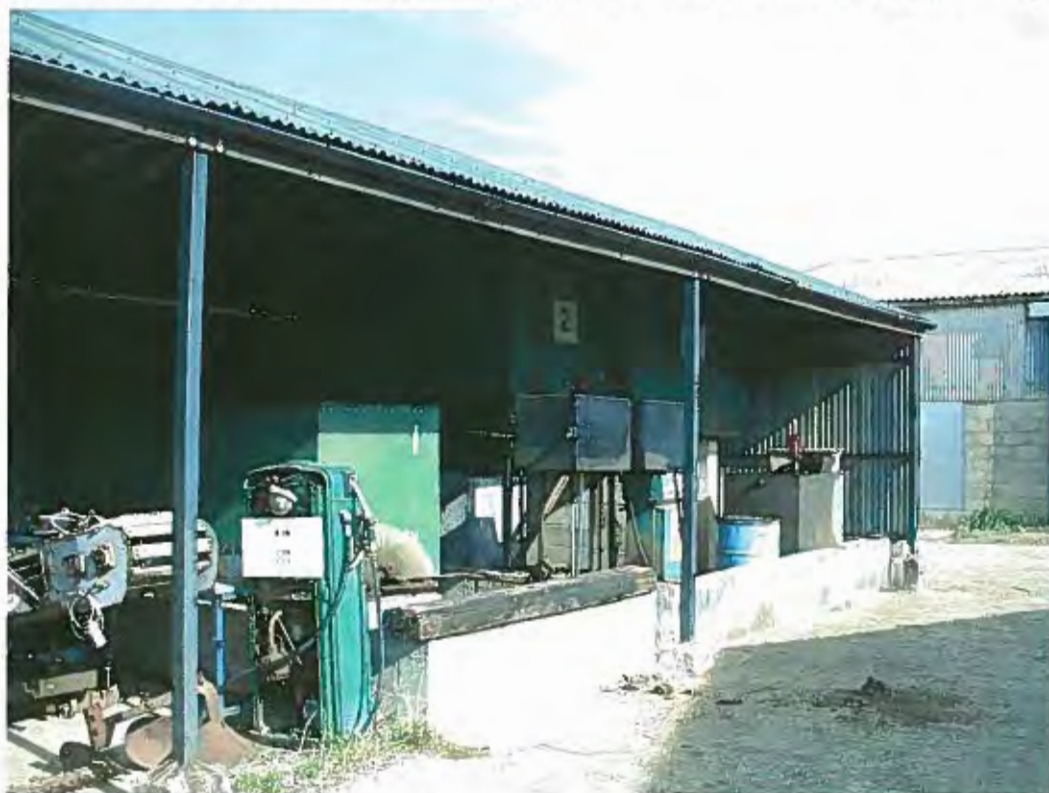
Redundant Tank 1 formally used to store white diesel and associated pump
