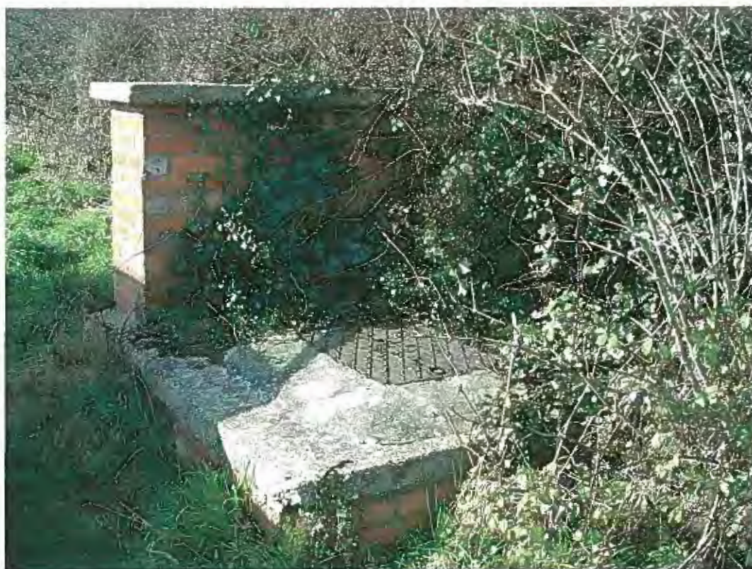
View on Borehole (NIAB Field).
