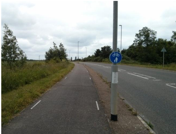
Photo 2.26 – Footway / Cycleway – Hatton’s Road
