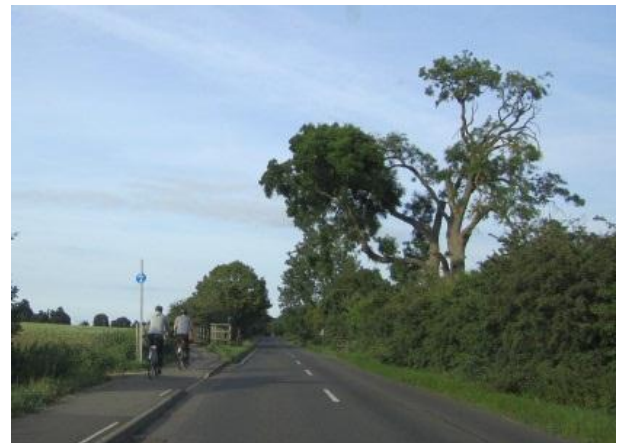
Photo 2.29 - Footway / Cycleway – Park Lane
