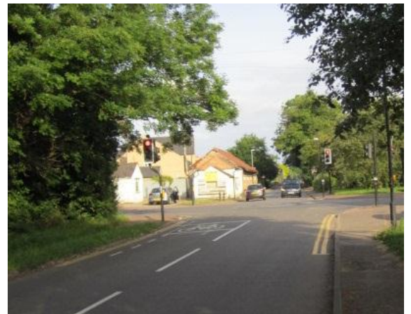
Photo 2.33 - Oakington Crossroads crossing (Cycle Route 24)
