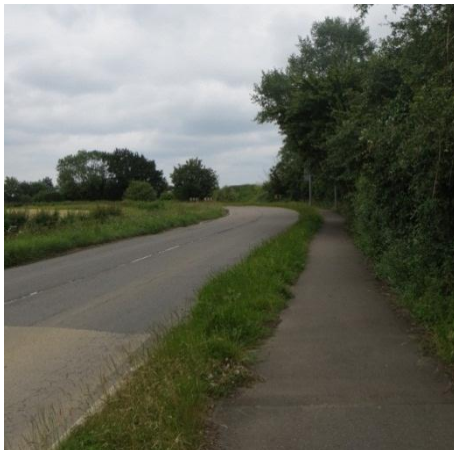
Photo 2.3 – B1050 Station Road
