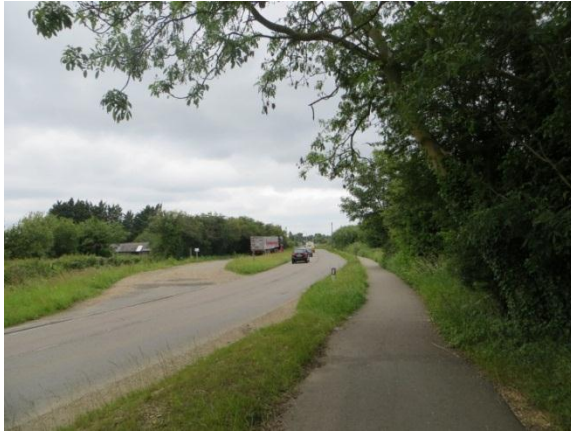
Photo 2.24 – Footway / Cycleway – B1050 Station Road
