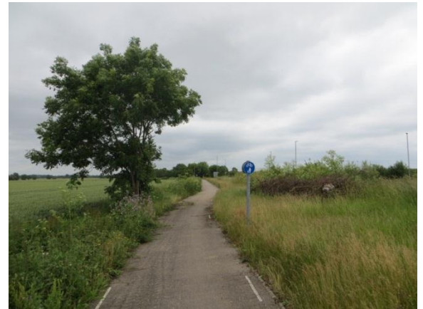
Photo 2.27 - Footway / Cycleway – Hatton’s Road
