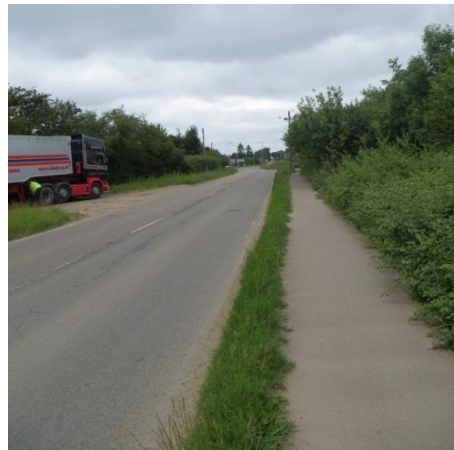
Photo 2.4 - B1050 Station Road
