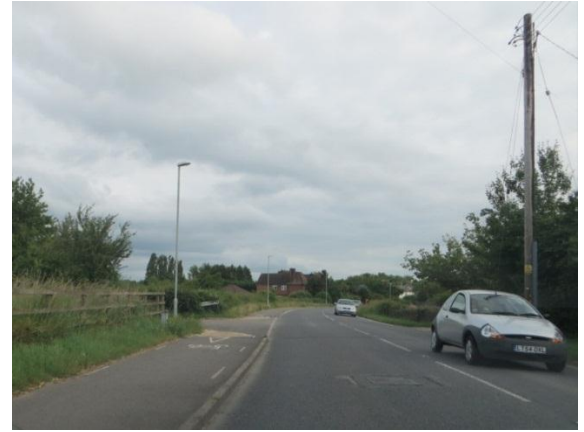
Photo 2.25 - Footway / Cycleway – B1050 Station Road
