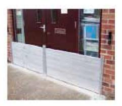
A flood-barrier is a secondary flood-proofing system to be used when the design elevation of the building is below the Base Flood Elevation. The purpose is to form a watertight seal in front of all building openings in order to prevent floodwaters from penetrating the structure.
