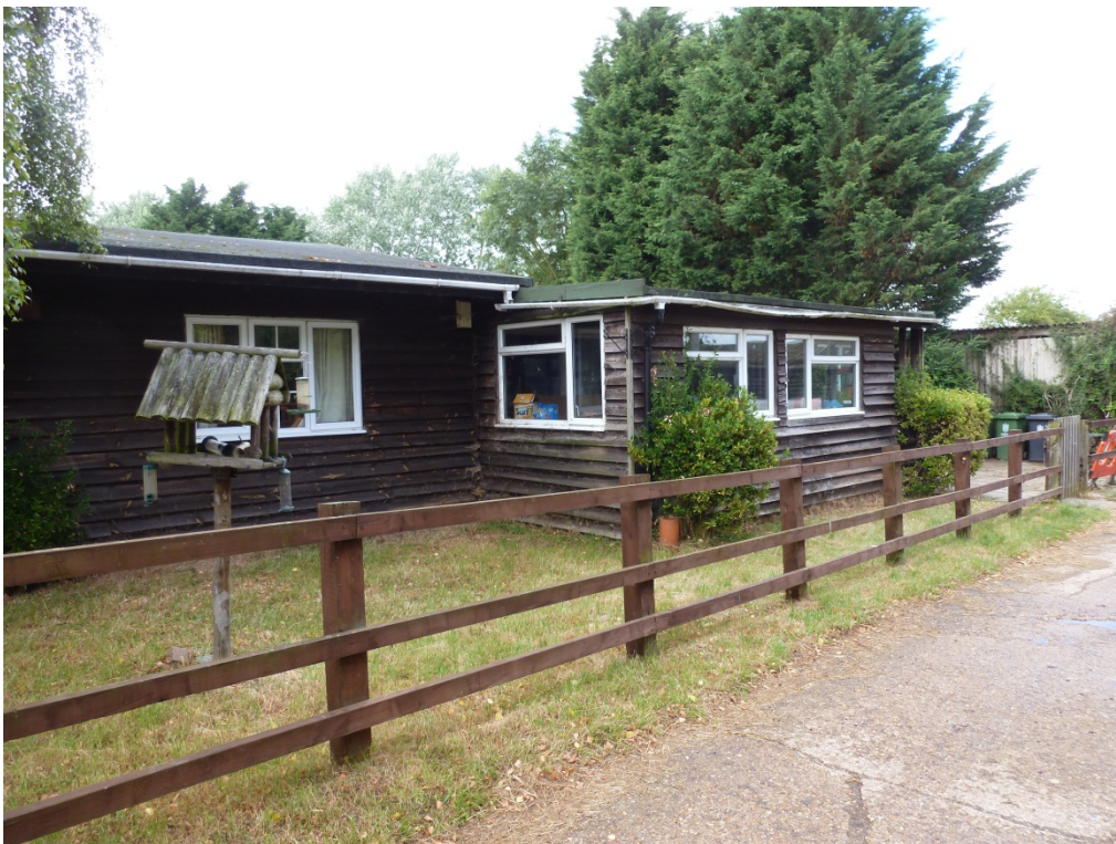
Photograph 2 B56, showing Pitched Roof Extension to the Southwest
