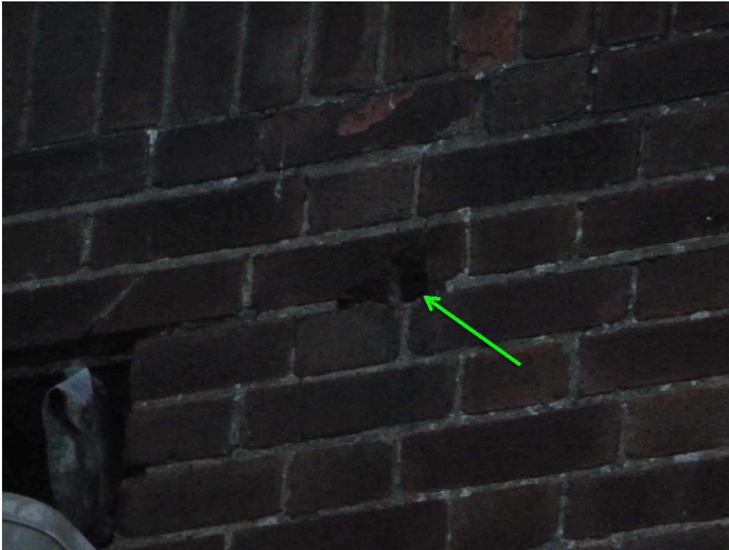
Photograph 3 Egress Location on Southeast façade of B2
