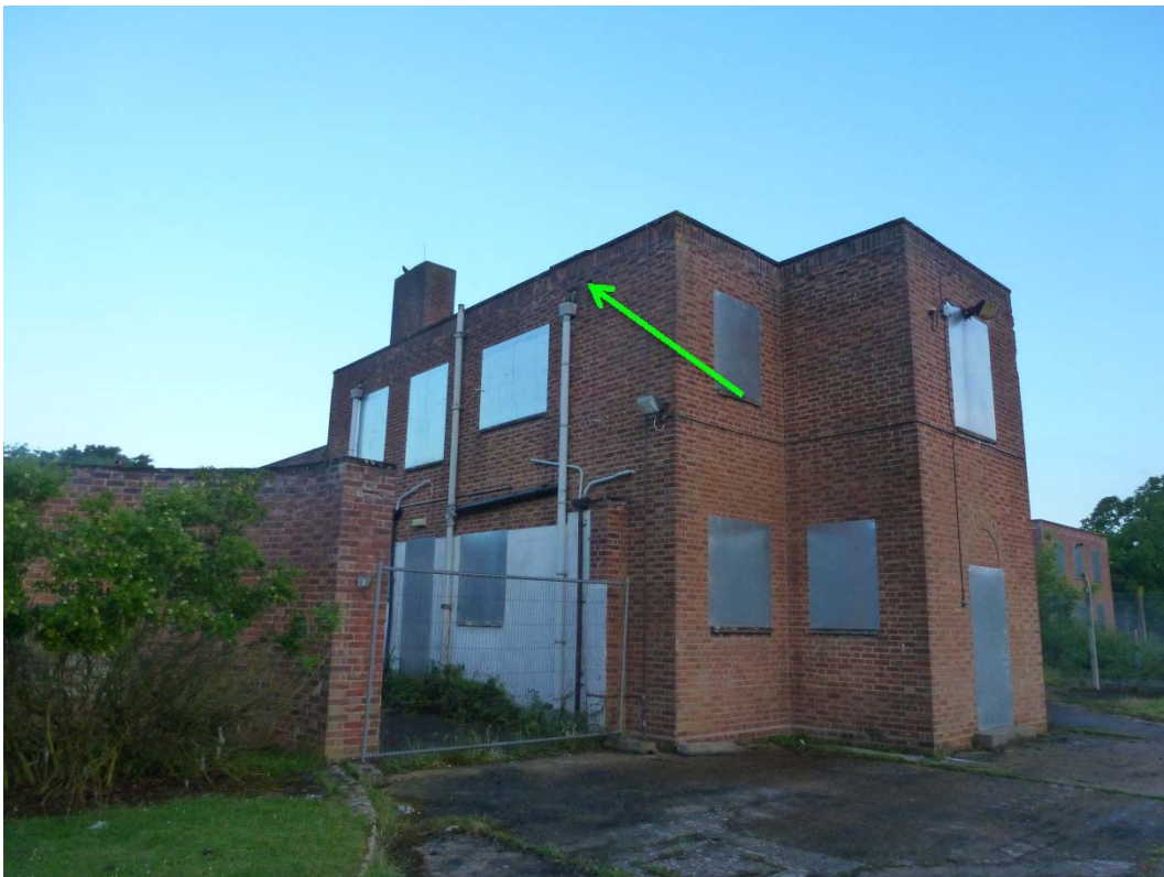
Photograph 4 Broad View of B2 and Egress Location
