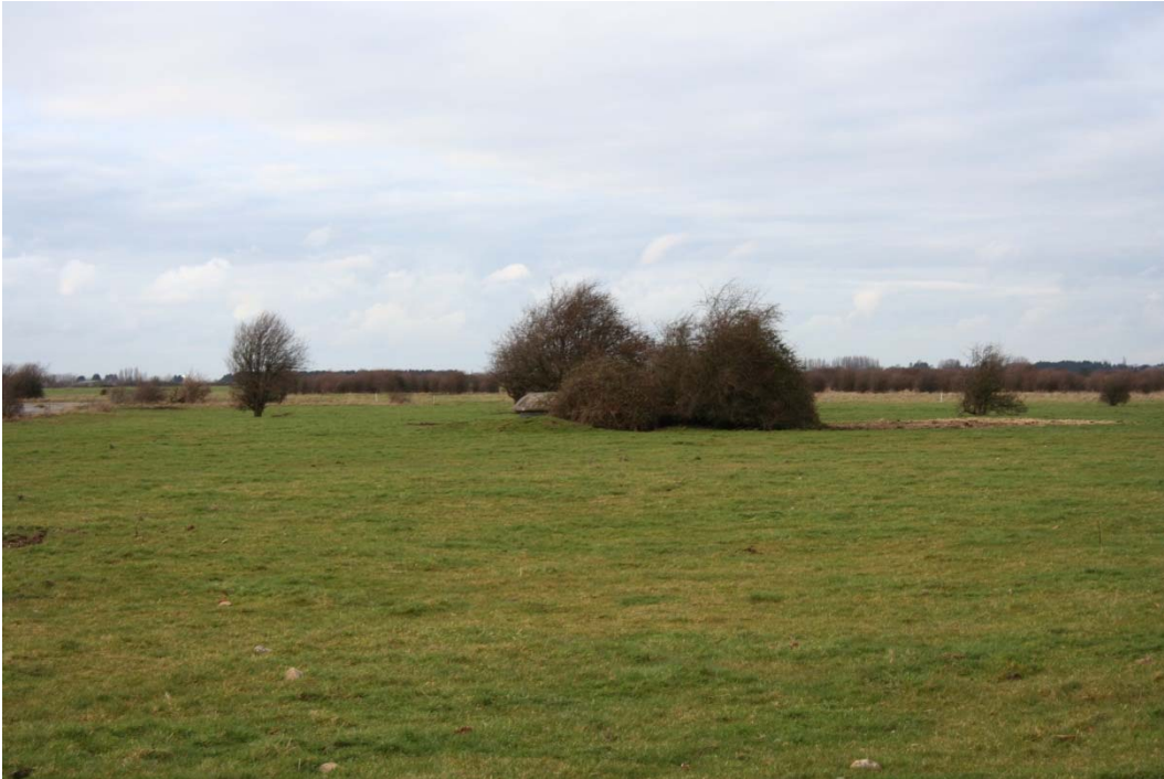
Photograph 9.4: Oakington-type pillbox 444 from the south.
