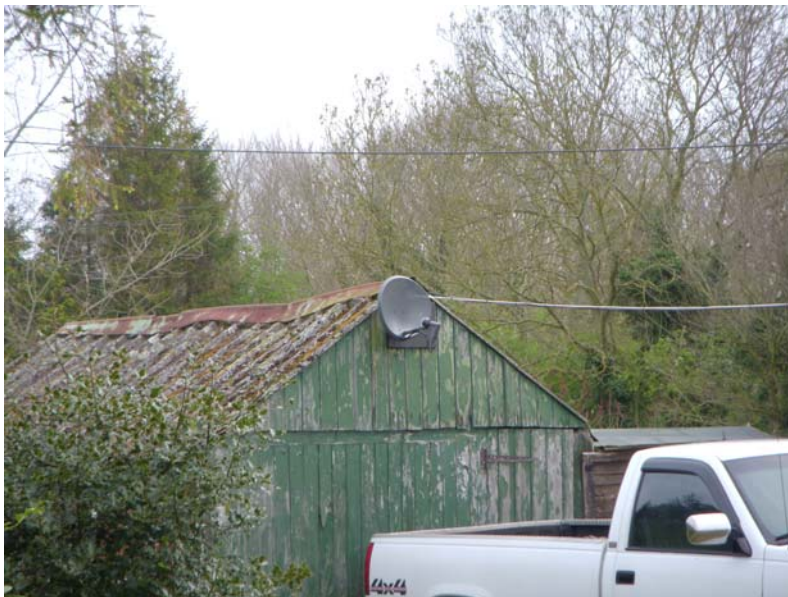
Satellite dish located on an outbuilding to avoid compromising the historic structure
