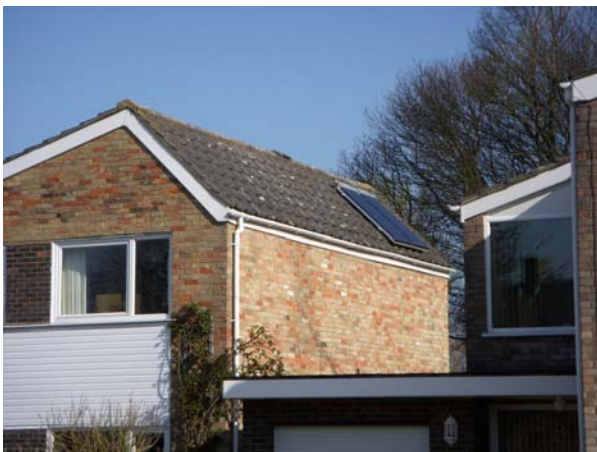
Discretely located solar panel on a side elevation of a 20 th century house in the Fulbourn Conservation Area
