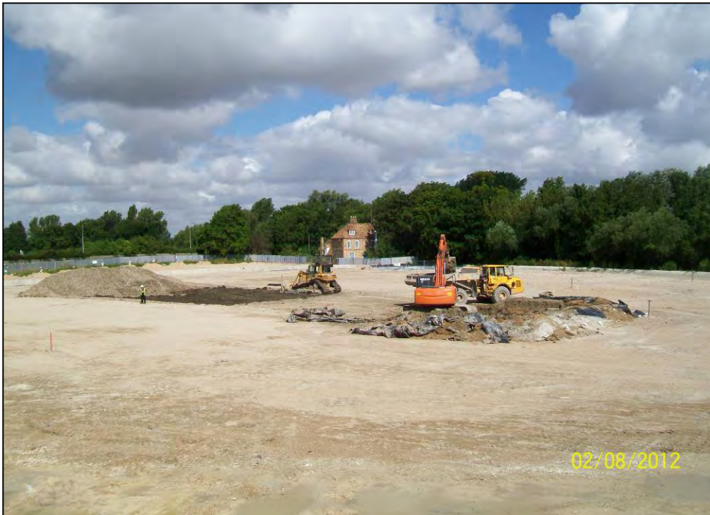
Figure 17. Final section of TB179 being reinstated.
