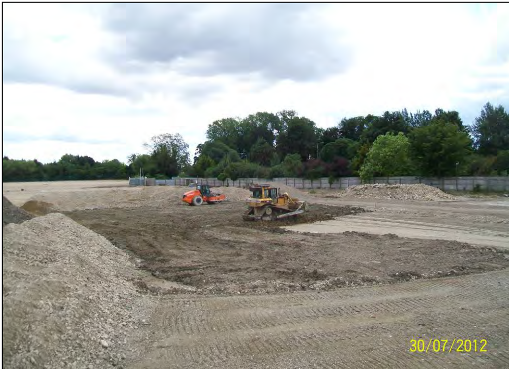
Figure 15. Caterpillar D6 laying down TB179 in single layer.
