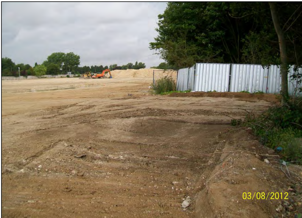
Figure 22. Reinstated off-site (B16) area with retaining bund around edge of reinstatement.
