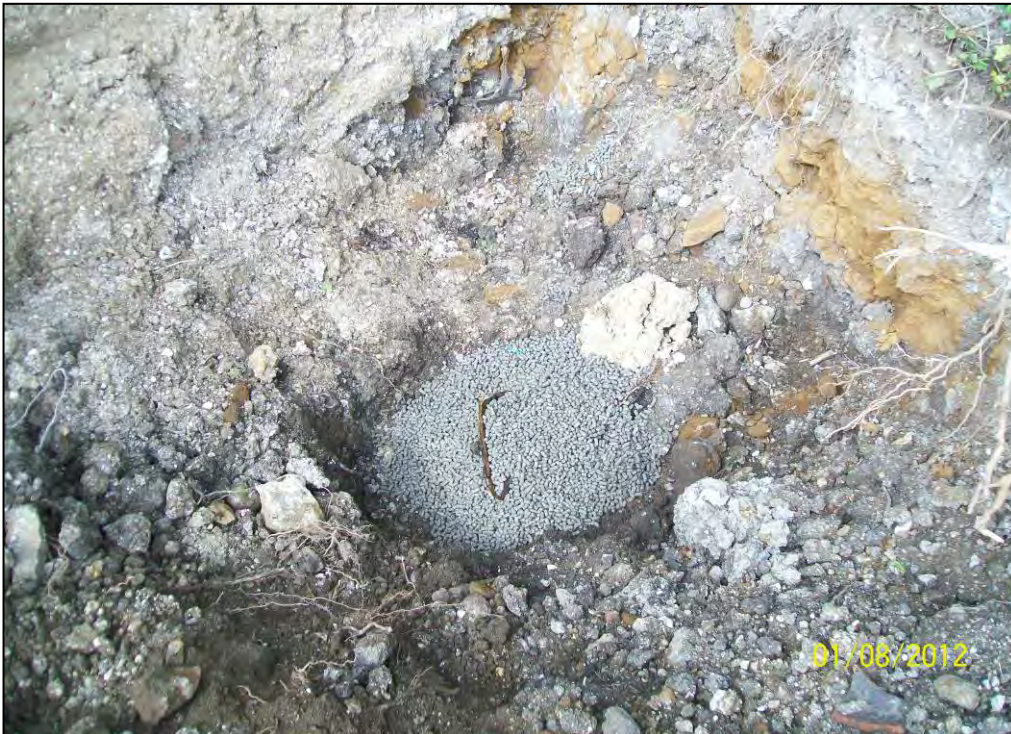
Figure 9. Steel pipe filled with bentonite prior to backfill in offsite area.
