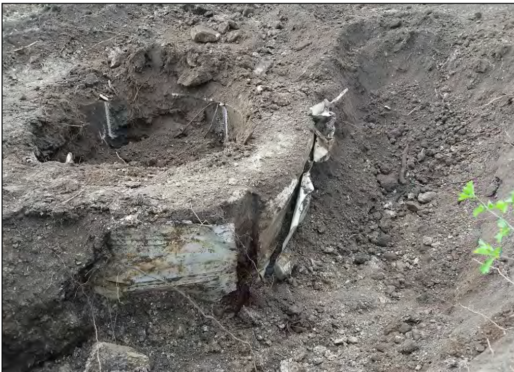
Figure 2. Manhole exposed by excavator during site investigation in March 2012.
