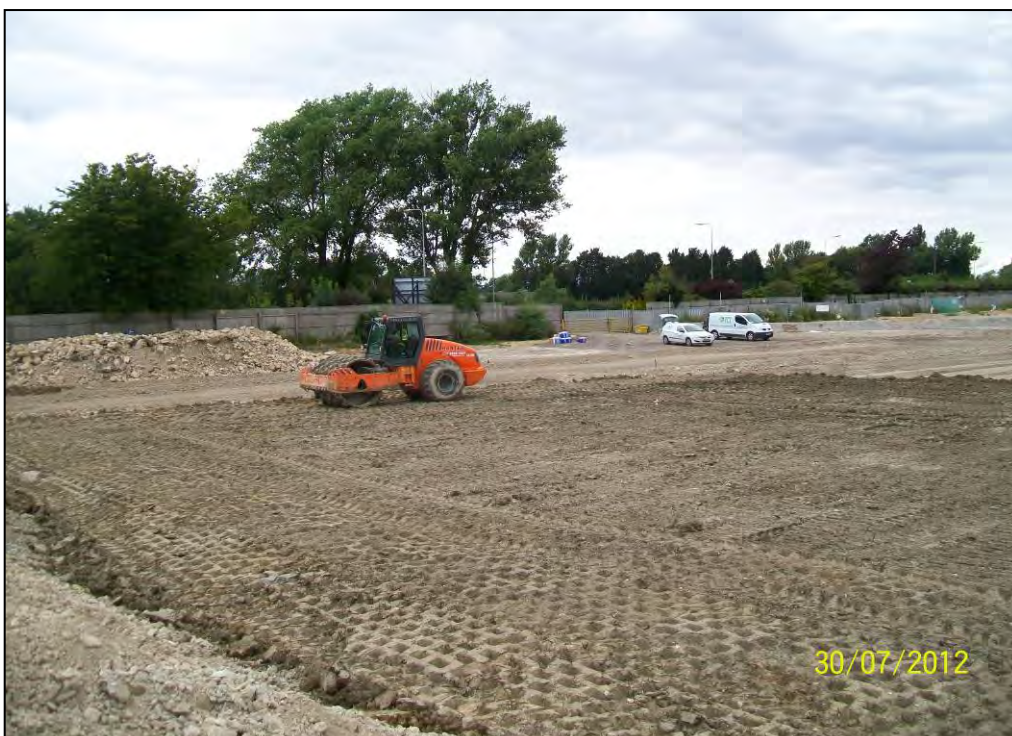
Figure 16. Sheep's foot roller compacting TB179.
