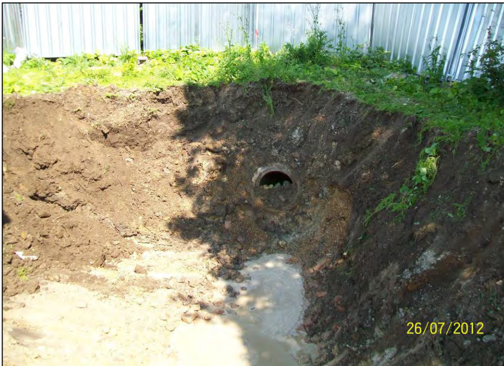
Figure 5. Manhole outfall excavated to site boundary.
