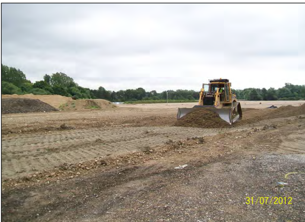
Figure 18. Caterpillar D6 reinstating crush concrete cap on top of TB179.
