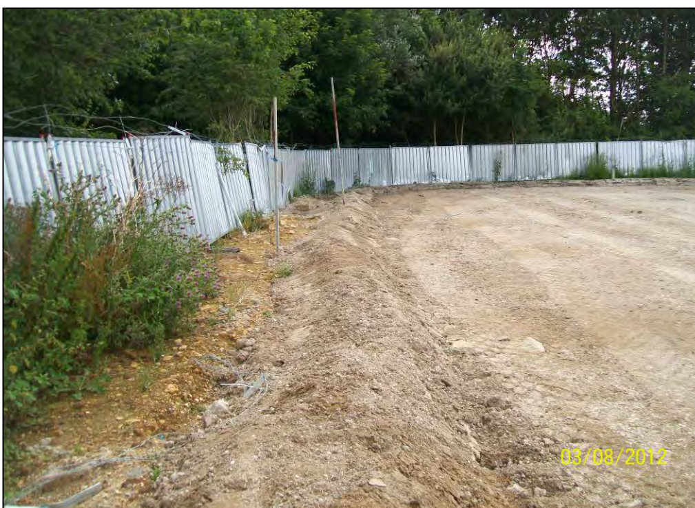
Figure 20. Retaining bund around reinstated material in A17, A18, B17, B18.
