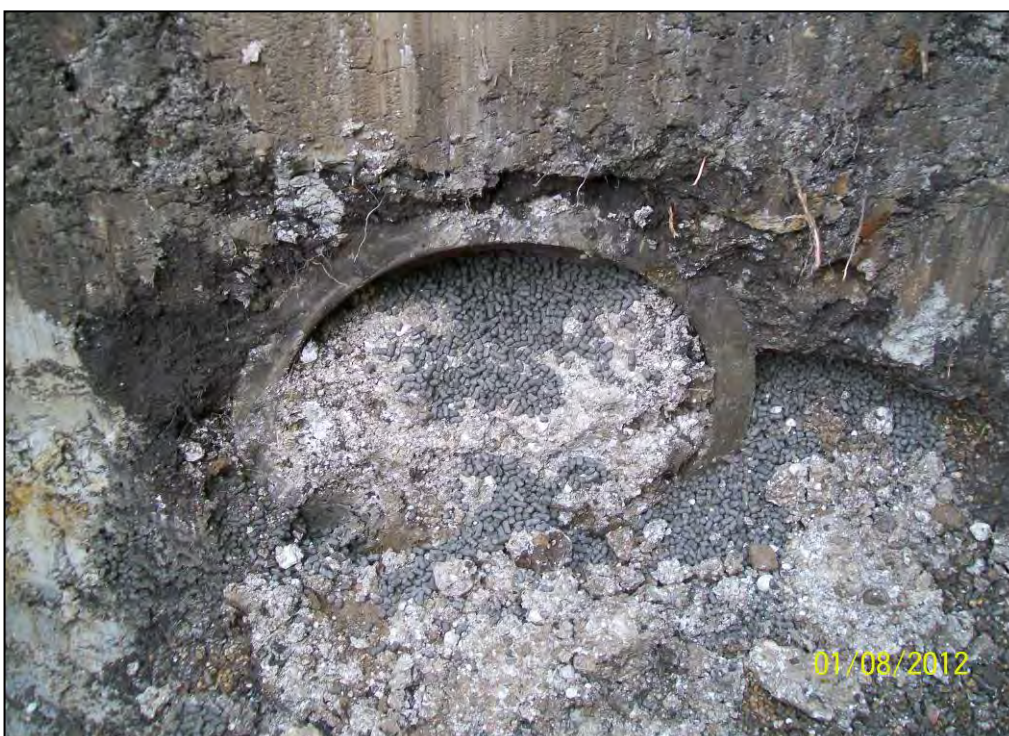
Figure 6. Manhole outfall fully filled with bentonite behind marl plug.
