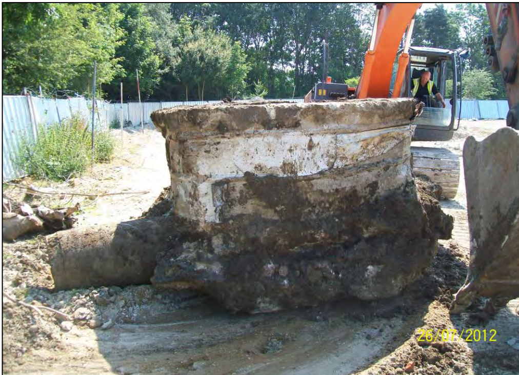
Figure 3. Manhole post excavation.
