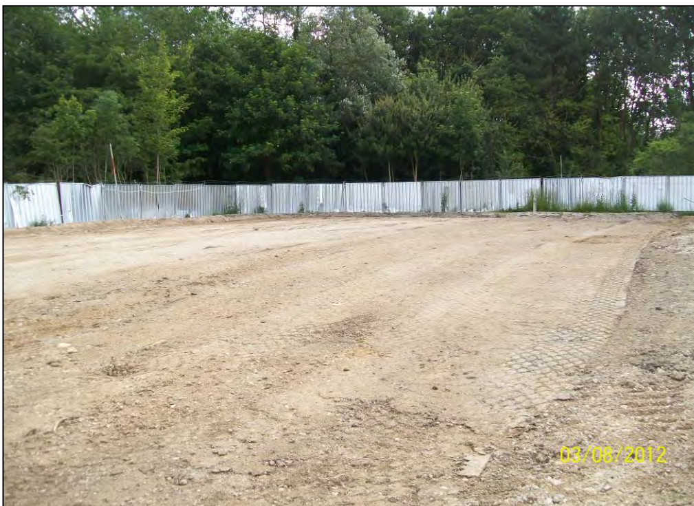
Figure 19. Zone 1 stockpile reinstated in grids A17, A18 B17, B18.
