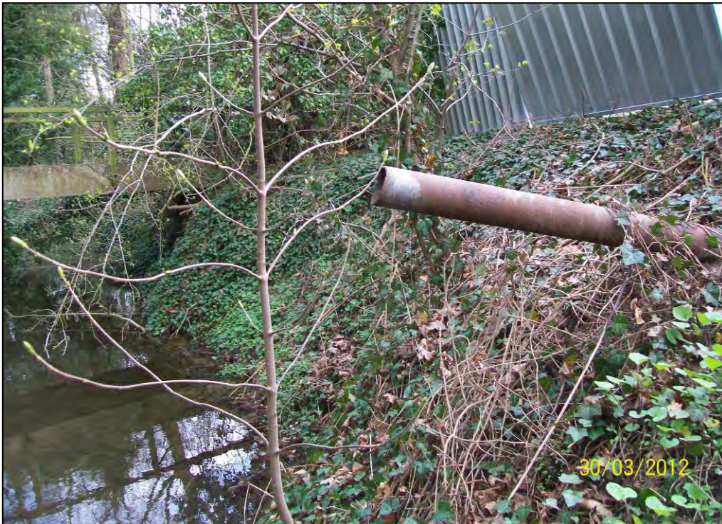
Figure 11. Close up of cast iron pipe.
