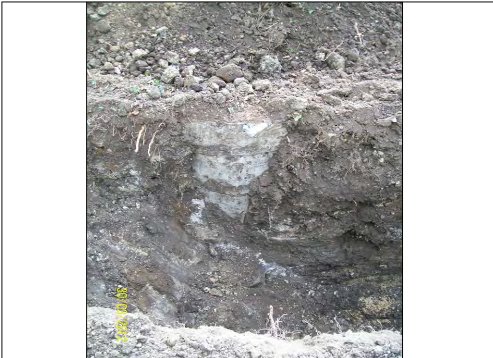
Figure 1. Manhole exposed in face of Trial Pit 2.
