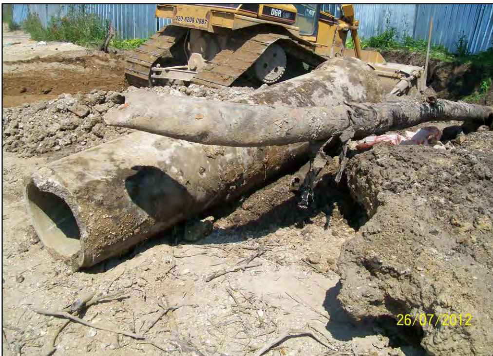
Figure 4. Manhole outfall pipe and excavated steel pipe.
