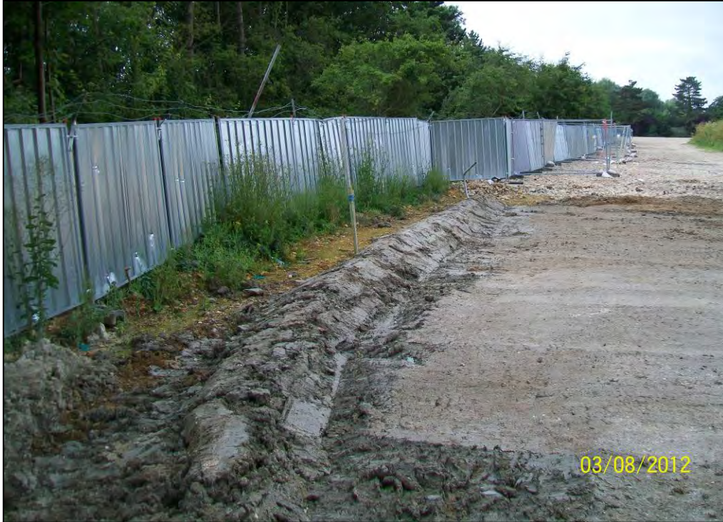
Figure 21. Retaining bund around reinstated material in A17, A18, B17, B18.
