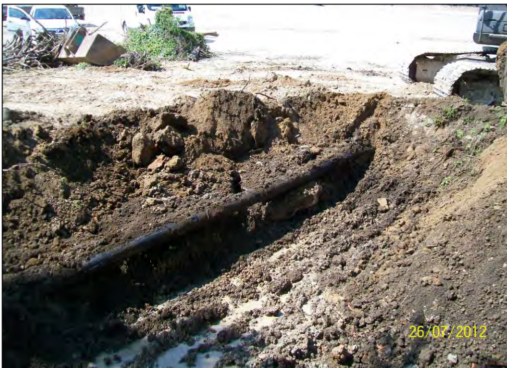
Figure 8. Steel pipe exposed in south face of excavation.
