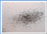
Mould spores growing on a ceiling
