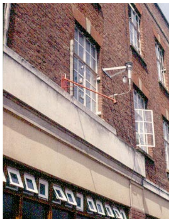
Monitoring in-takes, Regent Street
