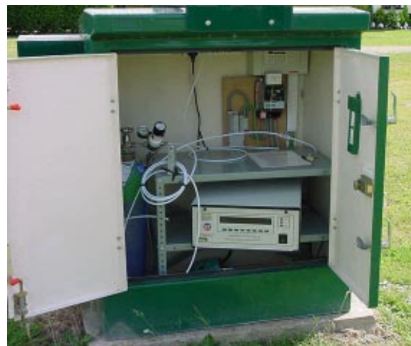
Sulphur Dioxide Monitor
