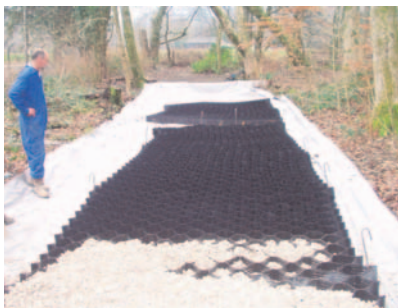
CellWeb during installation.
