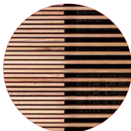
Slatted Timber Facade within Bronze Aluminum Vitrine Boxes
