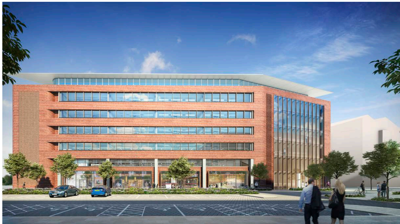
• Eastern View - Roof Canopy
