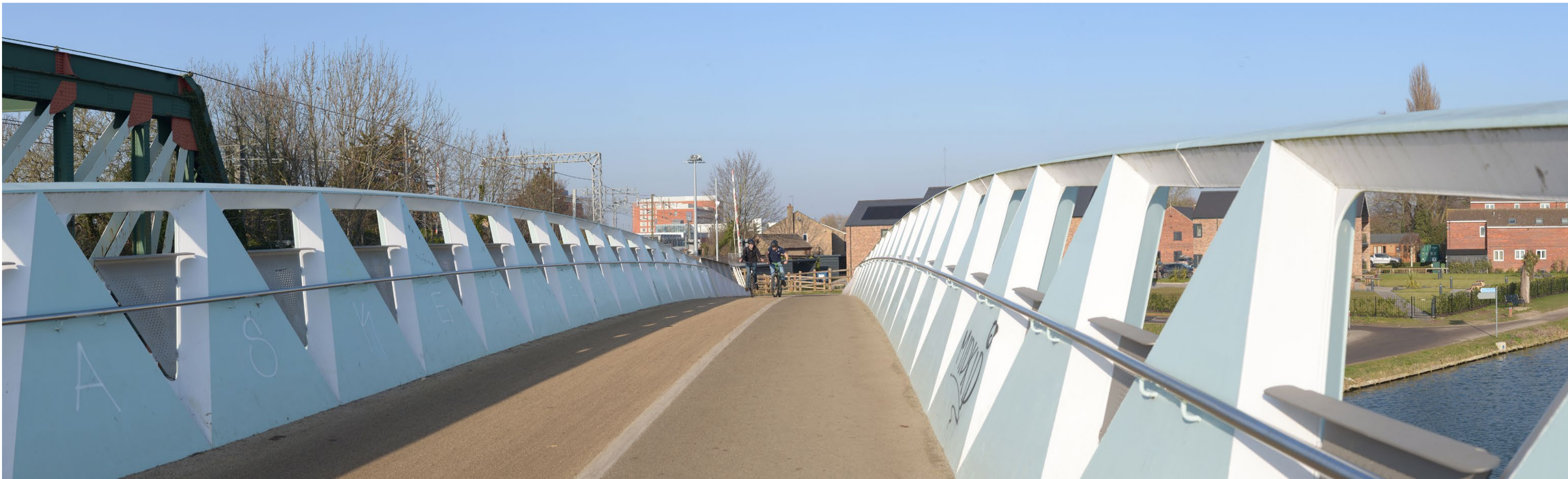
VIEWPOINT E1: CHISHOLM TRAIL BRIDGE ON RIVER CAM
