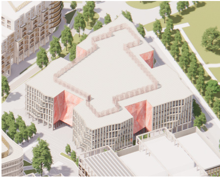
Fig. 164 Aerial View S9
