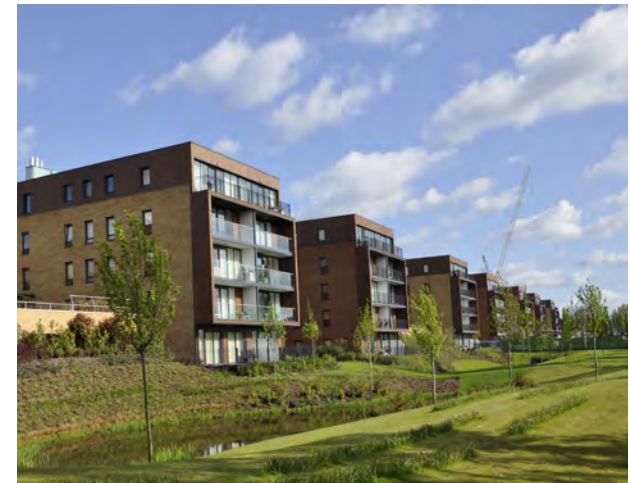
Residential flats overlooking park (Kidbrooke, Greenwich)
