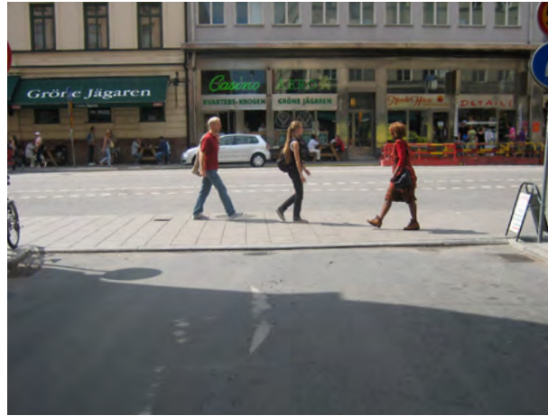
Example of a continuous footway across a side street, Stockholm
