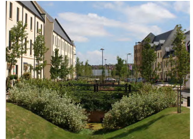
Example: Vegetated sustainable drainage watercourse in Upton, Northampton
