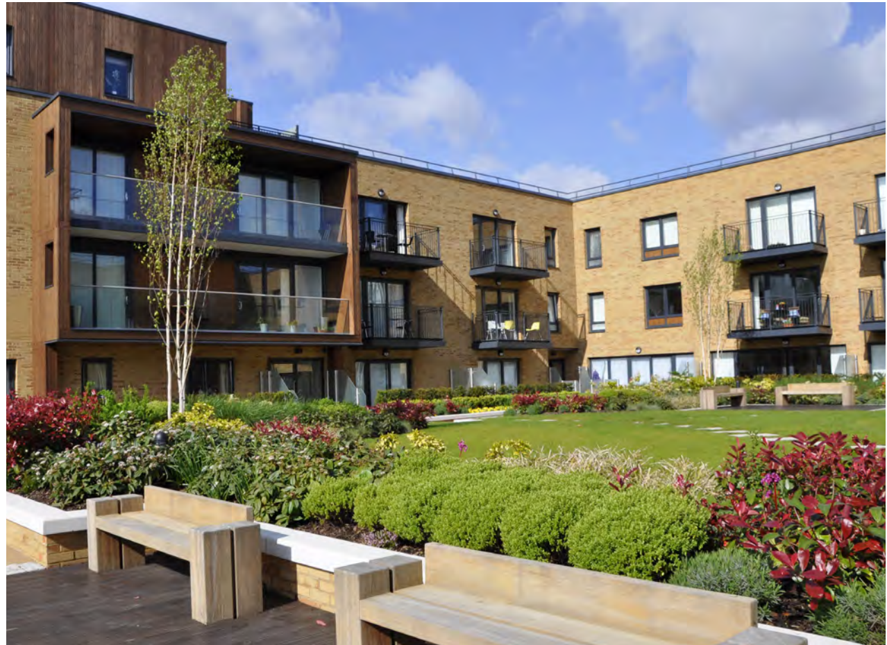
Smaller street blocks with communal courtyard over car park (example: Kidbrooke, Greenwich)
