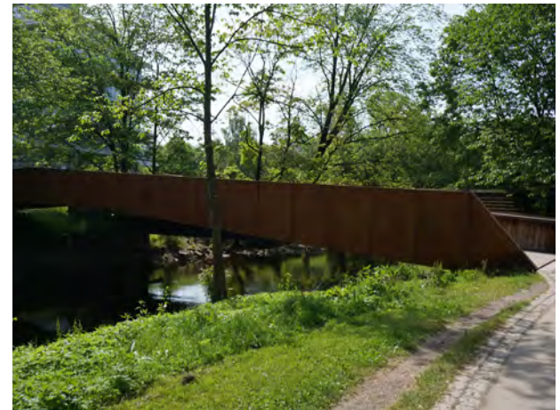
Frequent bridges connect across
