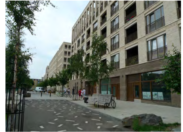
A creative public realm approach can be implemented with opportunity for play, Stoke Newington, London
