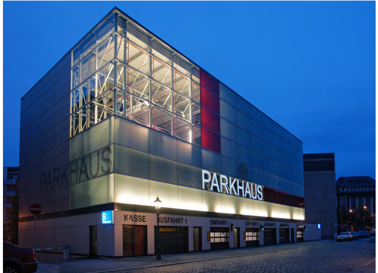
Example of a fully automated high capacity car park
