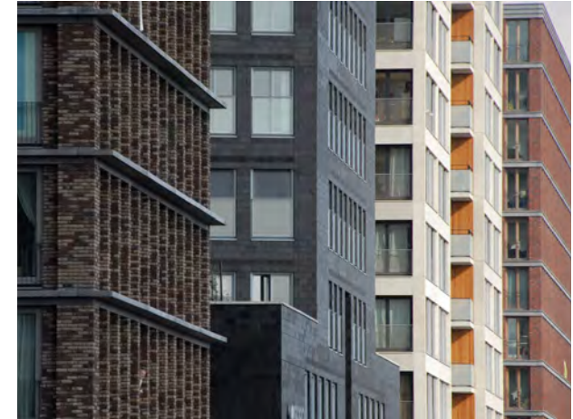
A range of muted natural colours, brick and masonry façades can create a varied yet coherent townscape (Amsterdam waterfront)
