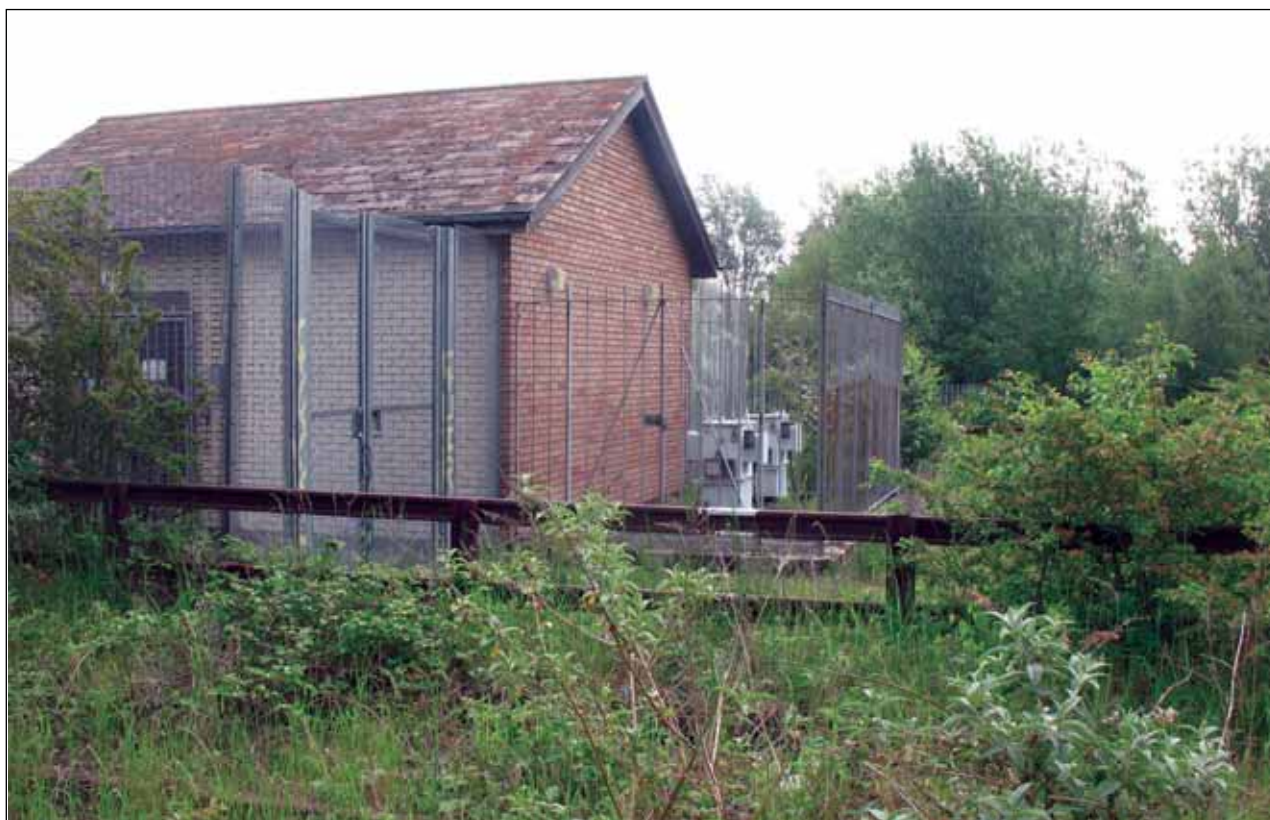
Plate 8: Existing Buildings – Generator Building
