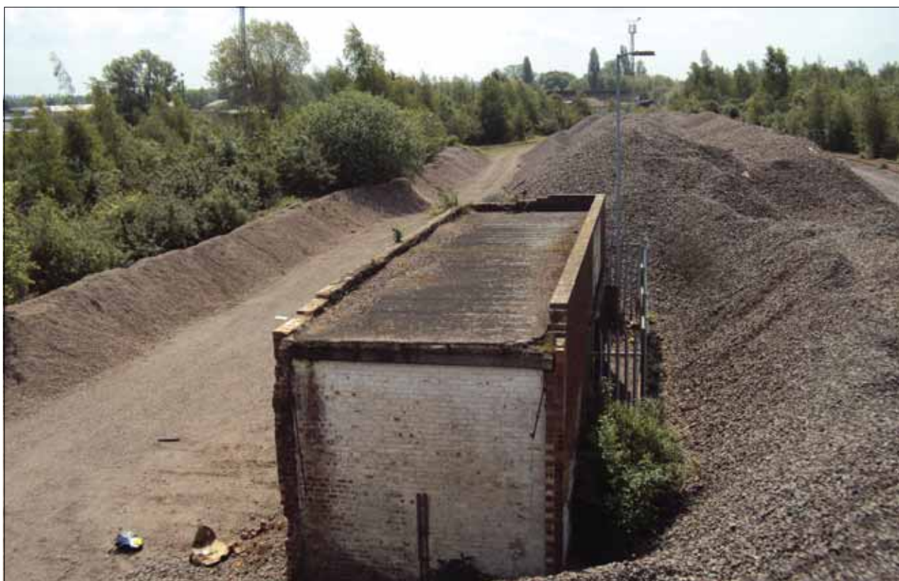
Plate 7: Existing Buildings - Sub-Station
