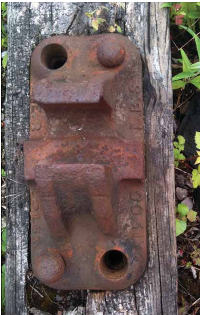
Plate 10: Railway Chair Baseplate (or tie plate)
