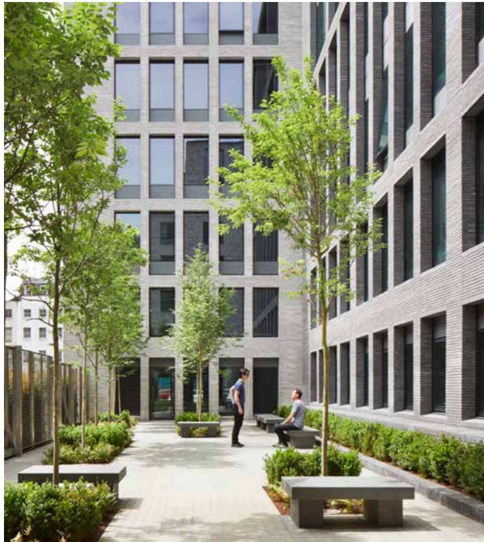
80 Charlotte Street, London - completed 2020
