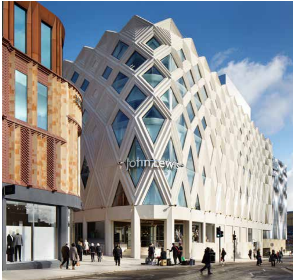
John Lewis Department Store, Leeds (UK) - completed 2017
