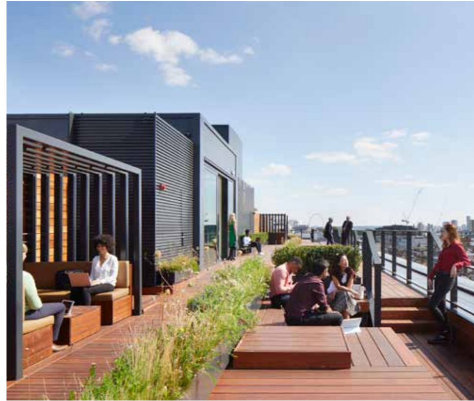
80 Charlotte Street, London - completed 2020
