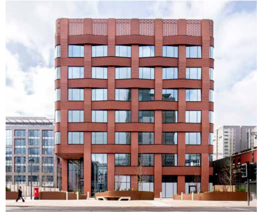
Three New Bailey, Salford - completed 2021
