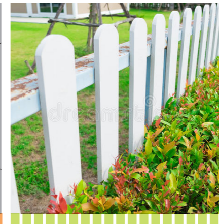
Picket fence - 1.2m high Timber picket fence to sensory garden, painted white with matching gates.
