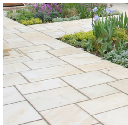
Shared terraces - High quality natural stone paviors
