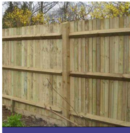
Close board fencing - 1.8m high close board timber fencing is proposed to form the boundary between adjacent residential properties. Painted dark green within the landscape buffer.
