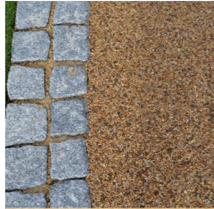
The Drive - Buff coloured bound surface with sett detailing
