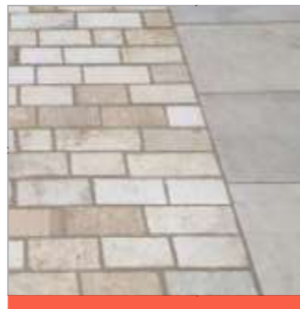
Entrance threshold - High quality natural stone large unit paviors with sett detailing to the edges
