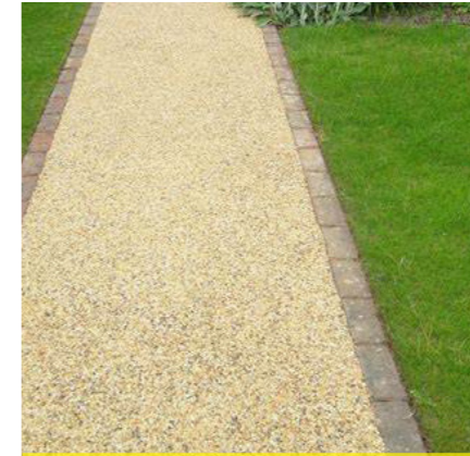
Primary / secondary pathways - Resin bound gravel pathway with brick edge
