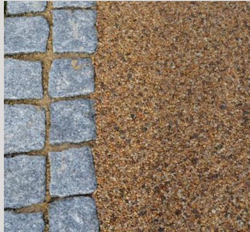
Coloured tarmac and granite edge detailing
