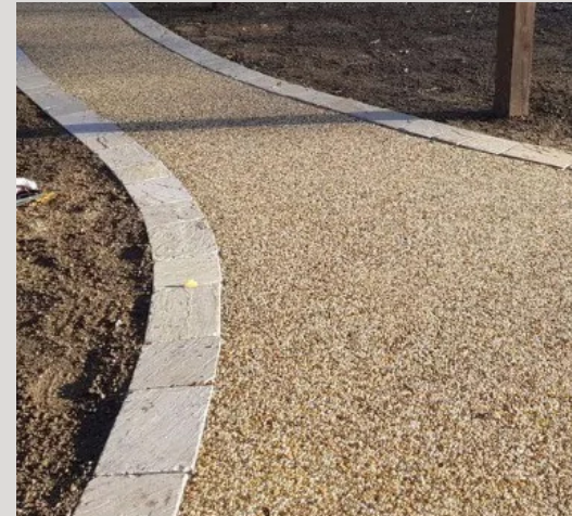
Buff resin bound gravel with brick or timber edge
