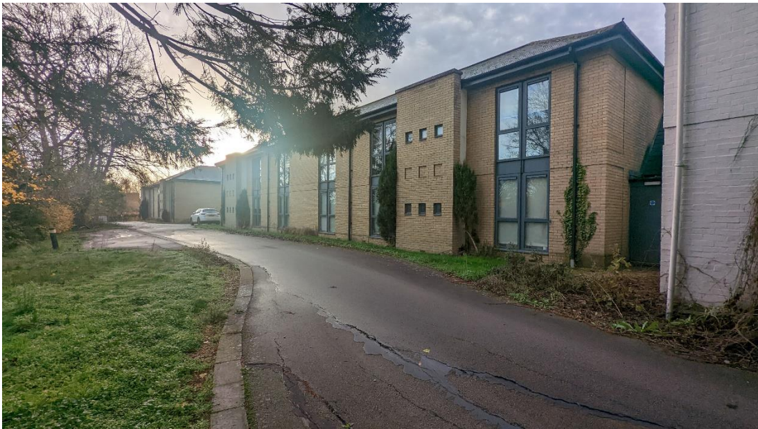
Figure 5 - Example of the modern accommodation blocks
