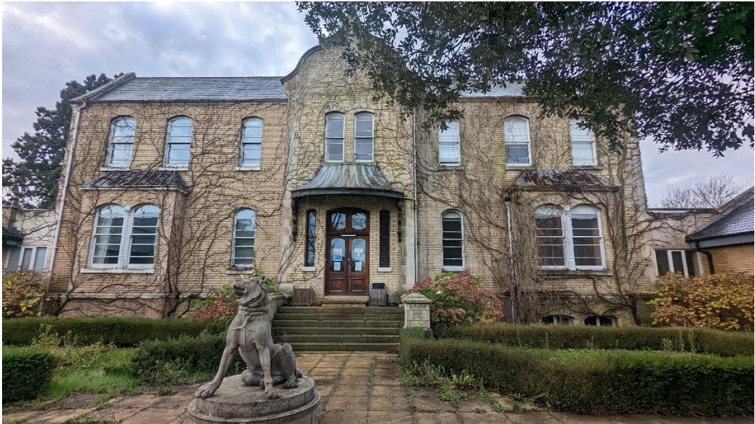
Figure 4 - Front elevation of the former Hotel Felix. The left-hand side is a modern extension which now creates a false sense of symmetry to this elevation. It obscures the original asymmetrical design of the building.
