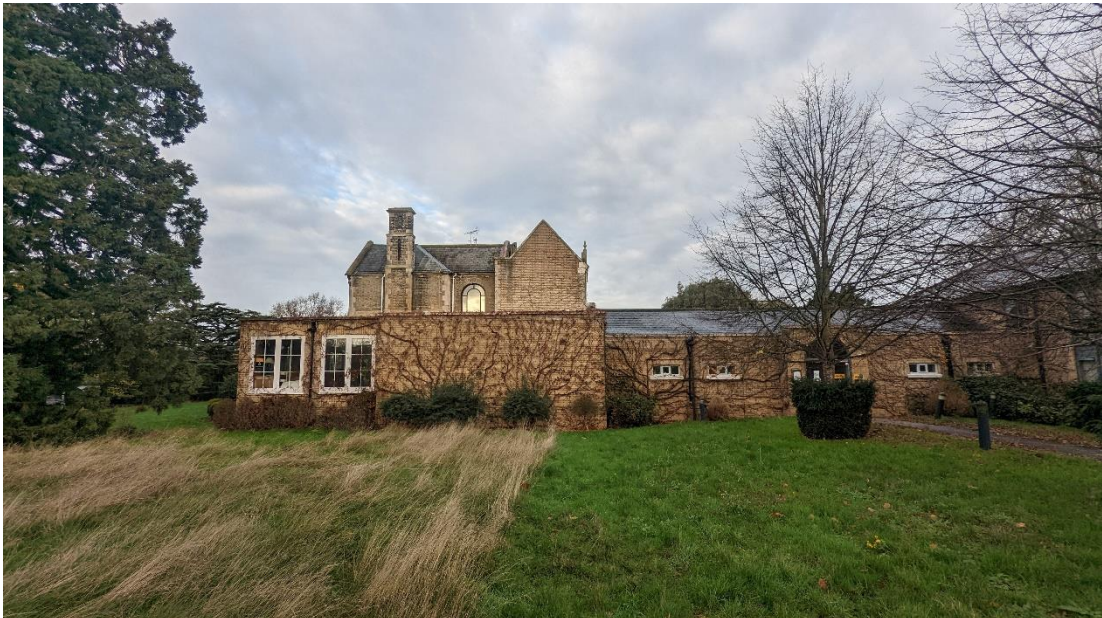
Figure 6 - View of the side of the orangery and one of the wings that have been added to the building. The right-hand side is a two-storey accommodation block, the appearance of which is shown in figure 5.
