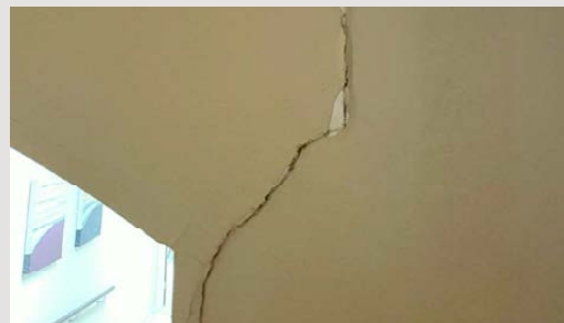
Substantial vertical crack to the side of the doorway.
