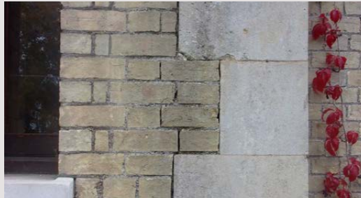
Vertical gaps starting to open on between masonry and stone quoins.
