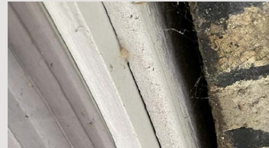
Significant movement of window frame and masonry
