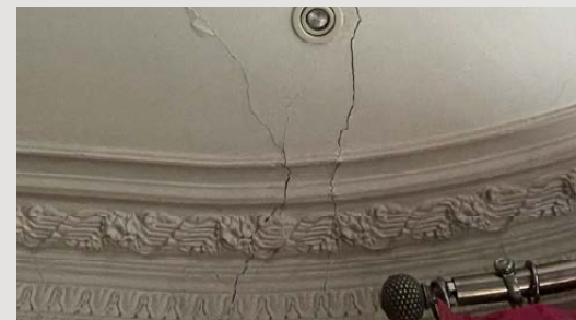
Cracking across ceiling to bay projection.
