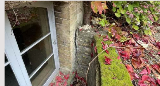
Large ivy root causing movement to lightwell below bay window.
