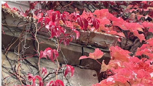
Movement and damage to stone work and guttering
