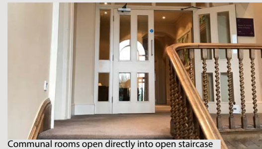
Communal rooms open directly into open staircase
