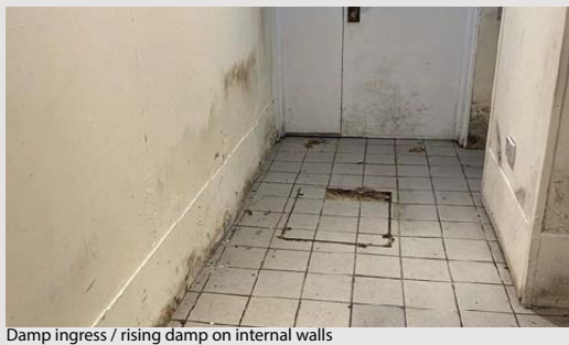
Damp ingress / rising damp on internal walls
