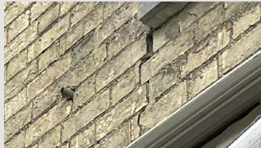
Cracking and dislocation to masonry below window
