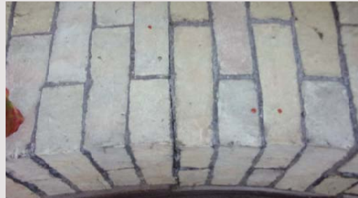
Several horizontal and vertical cracks in masonry.
