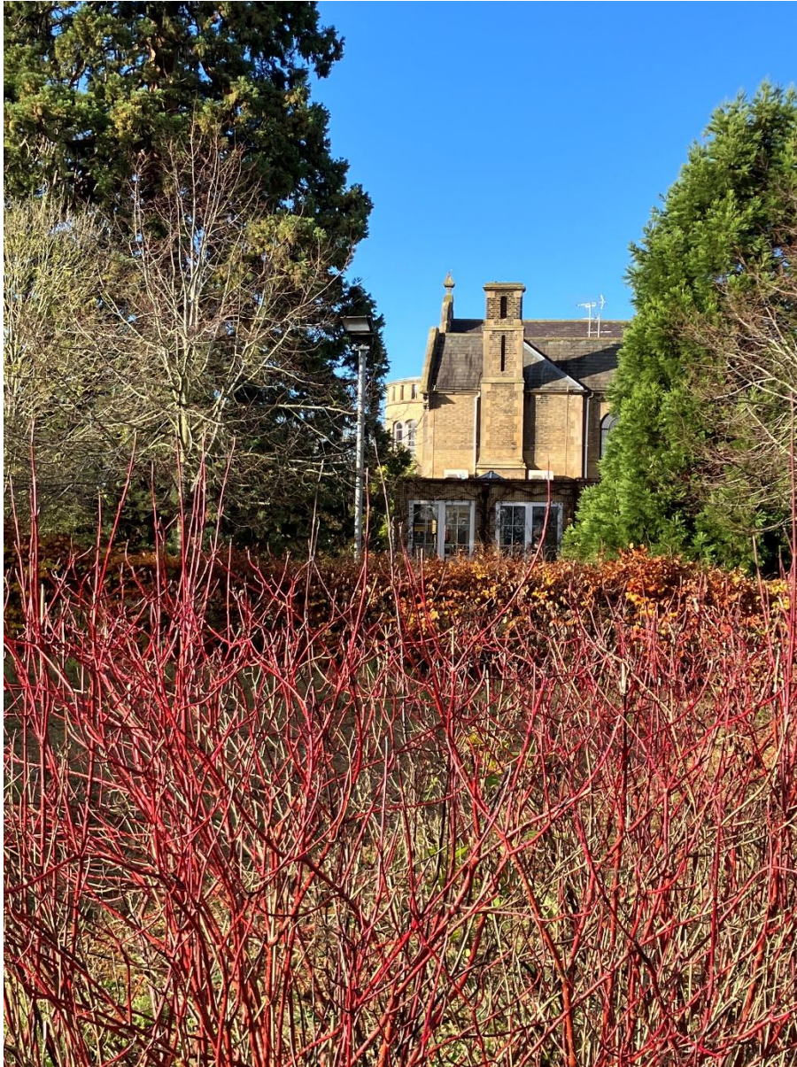
Figure 3 – Hotel Felix side elevation showing decorative chimneys and gable copings
