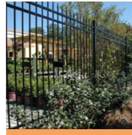
Metal railing - 1.8m high metal railing painted black forming the secure edge between the garden spaces and arrival courtyard, with matching metal gate.
