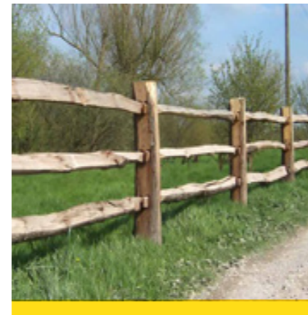
Chestnut cleft fencing - 1.2m high Chestnut cleft timber fencing enclosing the east of the site.
