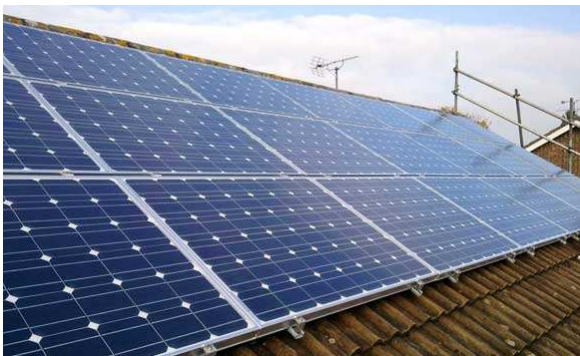
Picture 1: Frame mounted PV on a flat roof
