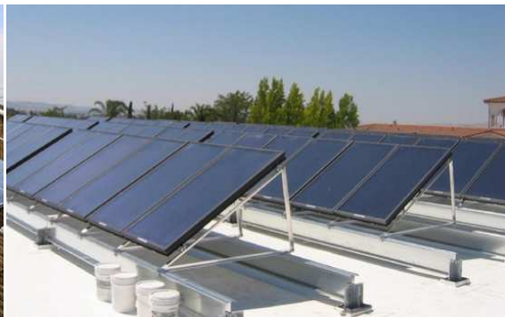
Picture 2: Roof Mounted PV Panels
