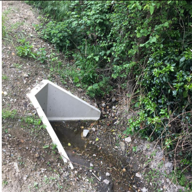
EXISTING HEADWALL FROM S106 SEWER
