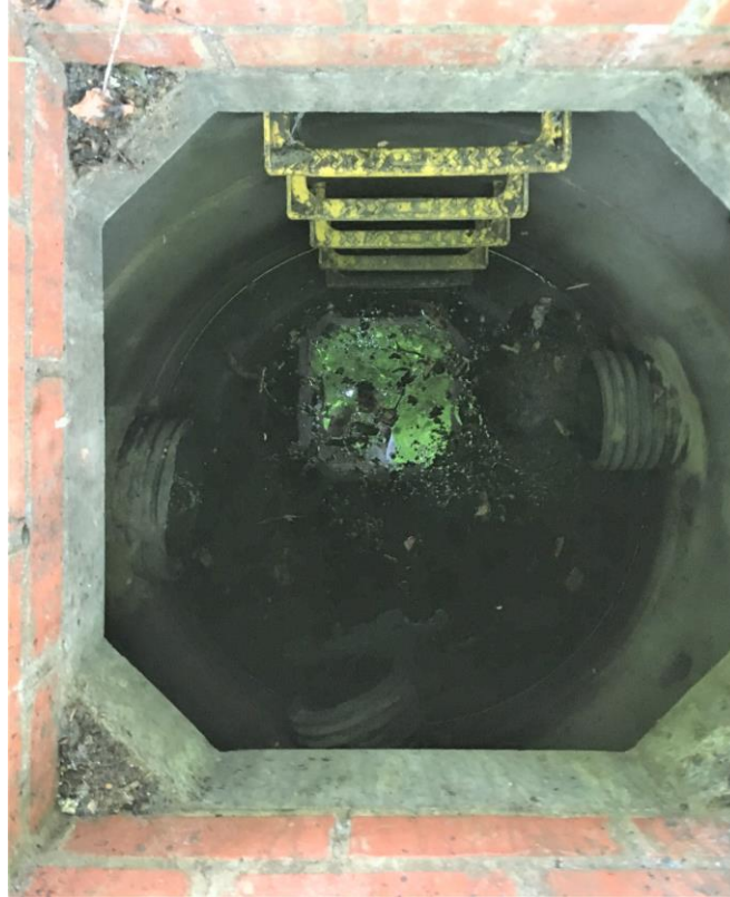
EXISTING SW MH 10 (Inlets 3 o'clock and 6 o'clock, outfall at 9 o'clock)
