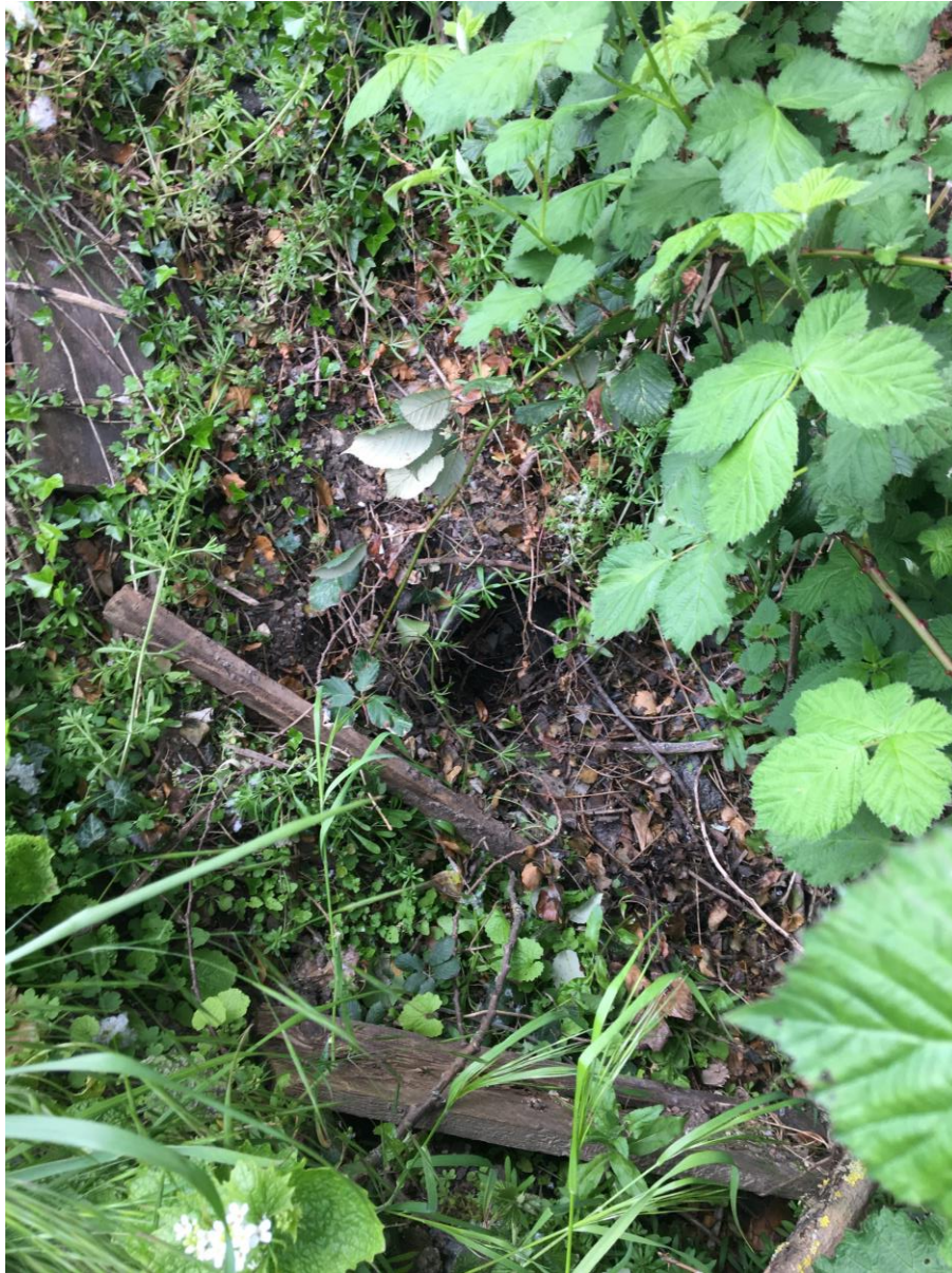
300mm DIAMETER OUTLET FROM SITE
