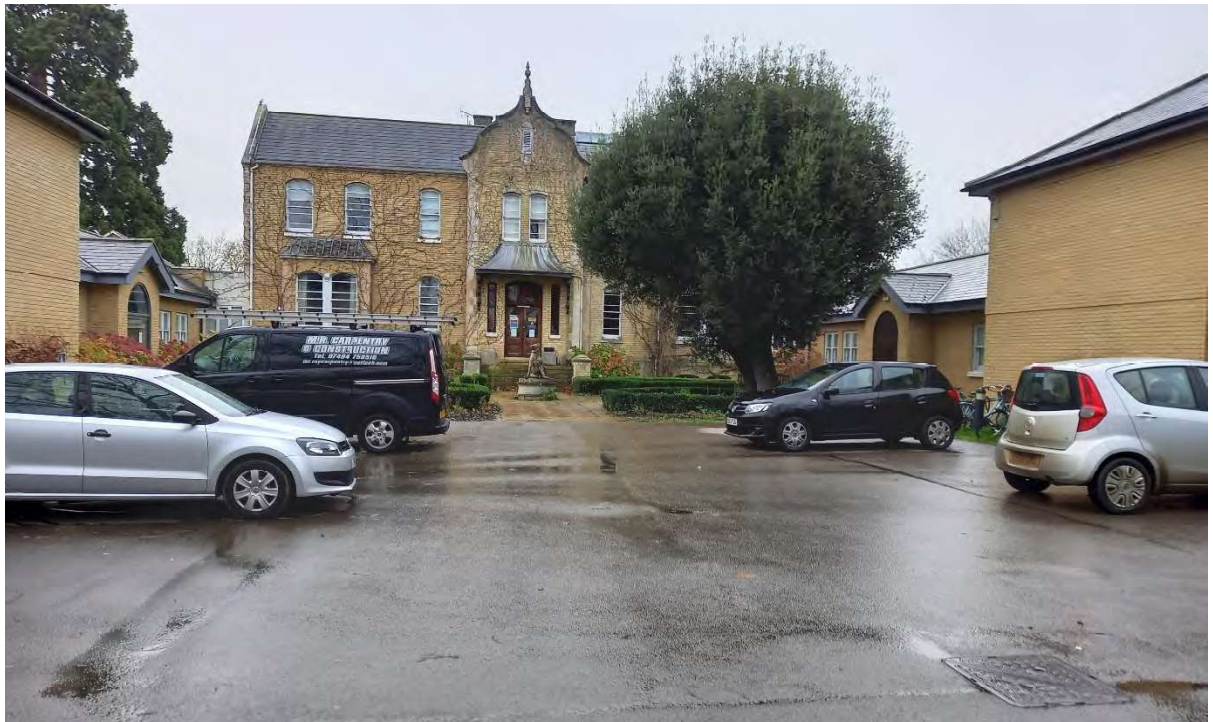
Figure 6: Existing hotel in centre of site, facing southwest.
