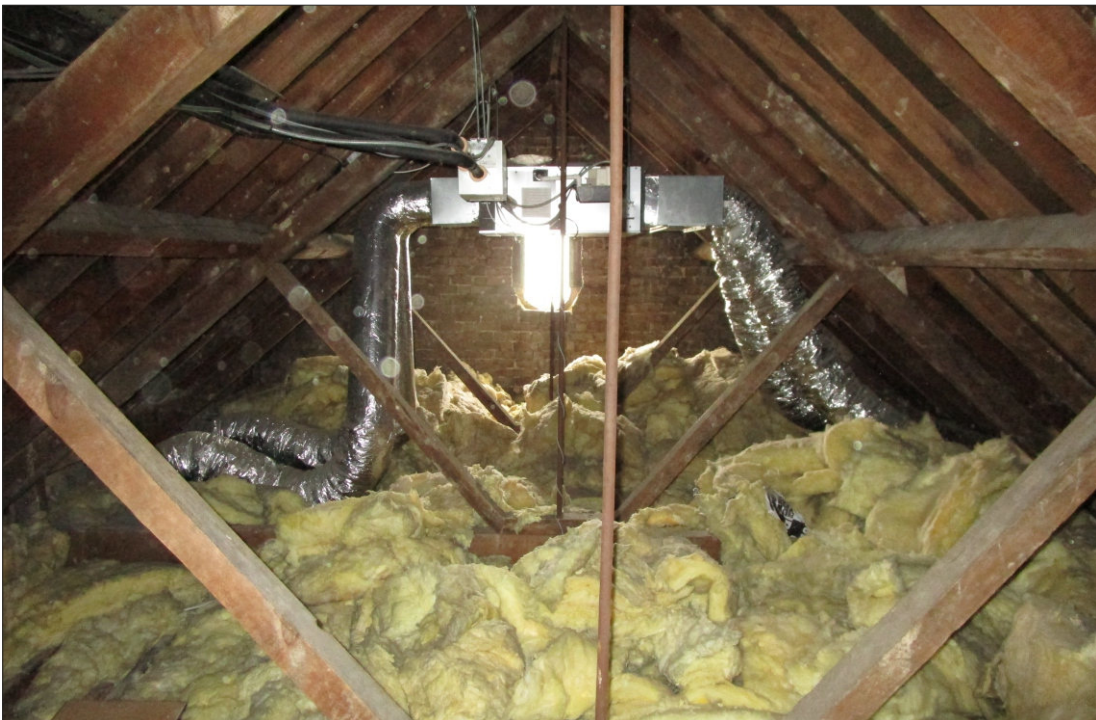
PHOTOGRAPH 8: Loft void within Building B1
