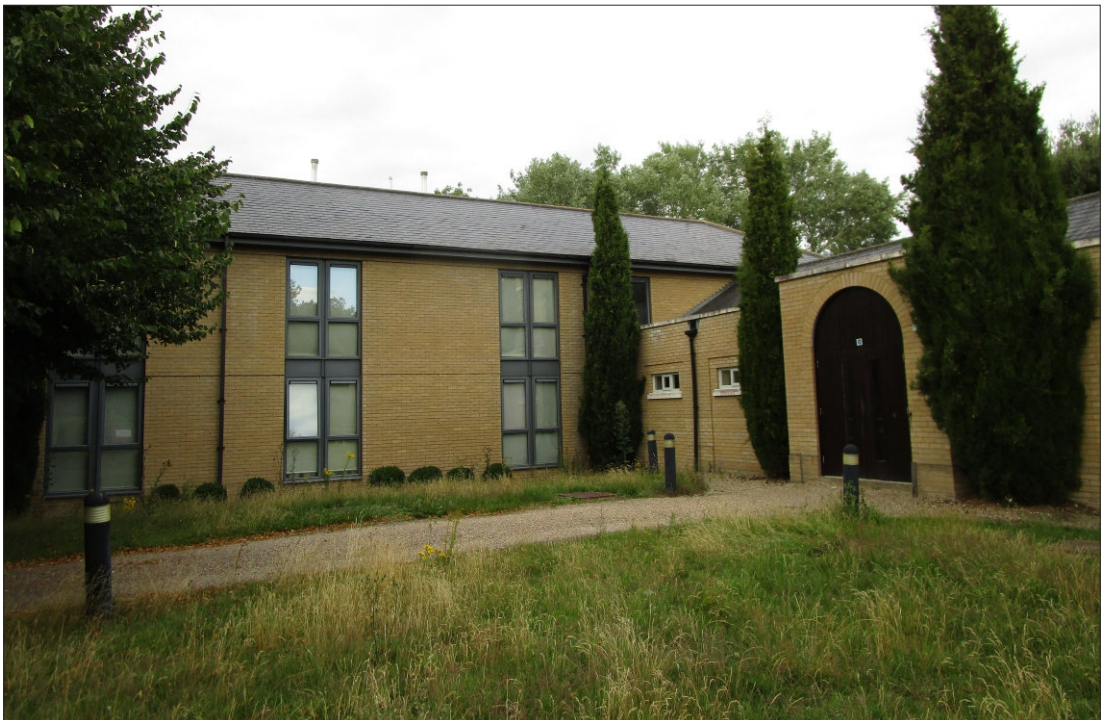
PHOTOGRAPH 2: Building B1, modern extension
