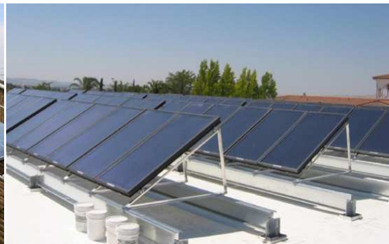
Picture 2: Roof Mounted PV Panels
