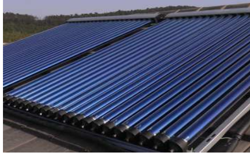
Picture 3: Evacuated tube solar thermal panels
