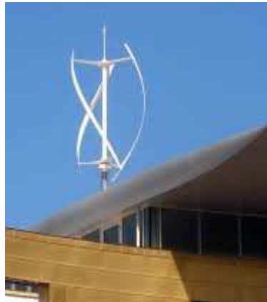
Picture 4: Micro-Wind Turbine (multiple required for reasonable yield)
