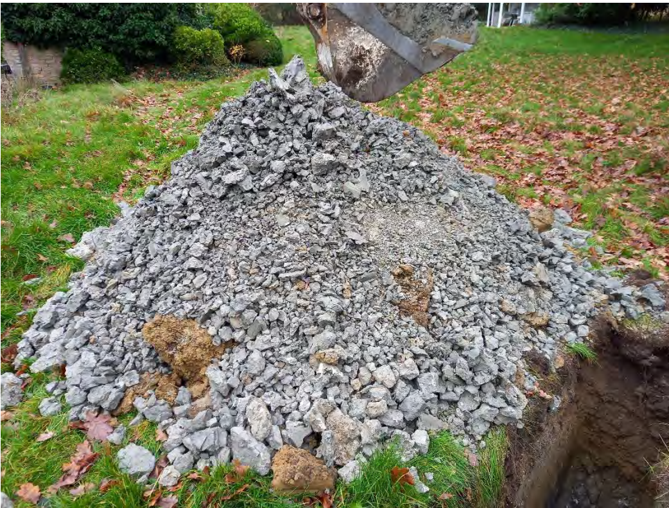
Photo 8: View of TP4 spoil.
