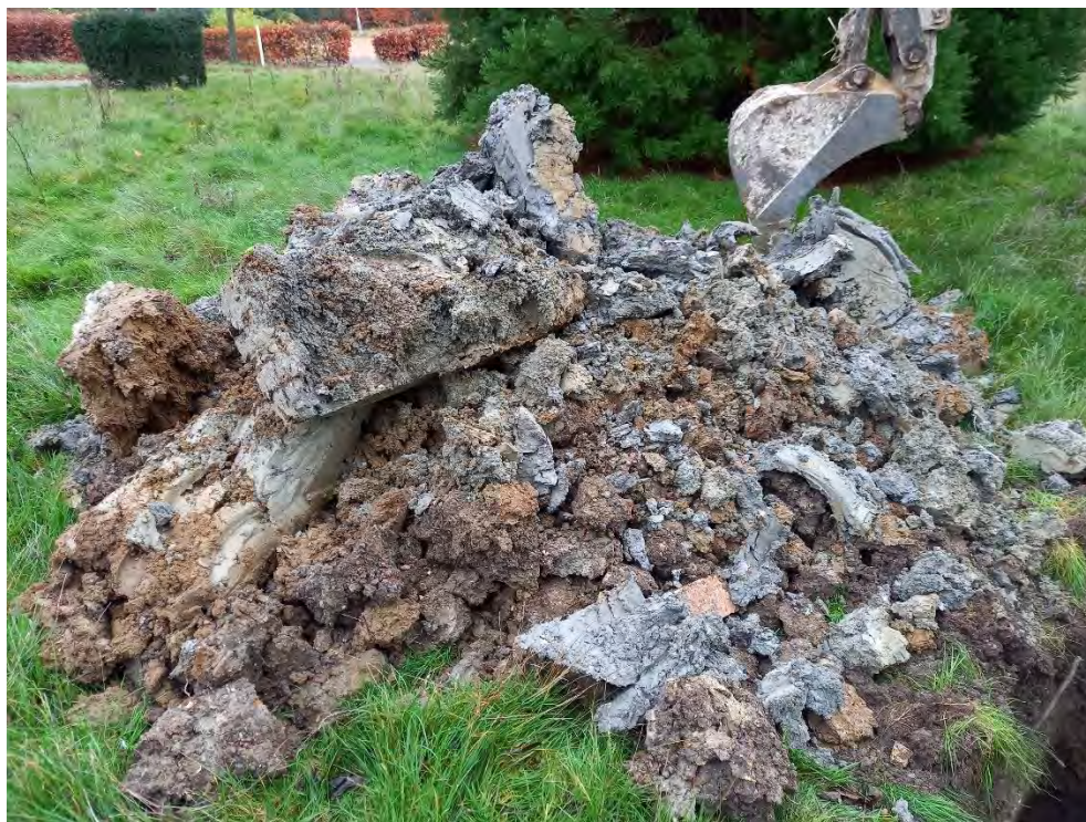
Photo 12: View of TP6 spoil.
