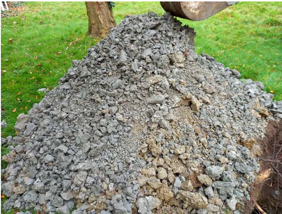
Photo 16: View of TP8 spoil.
