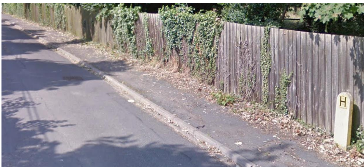
Footway Flanking Whitehouse Lane
