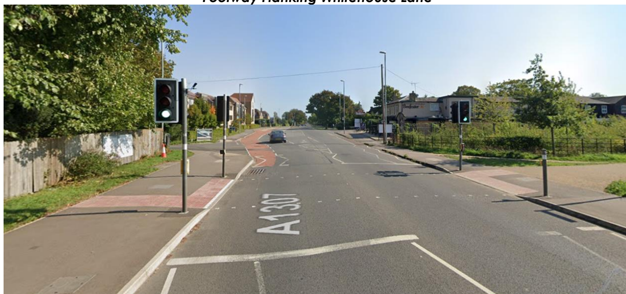
Signal Controlled Pedestrian Crossing on A1307
