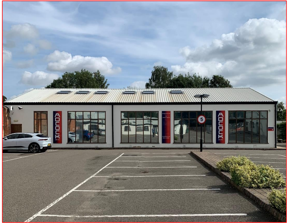
Plate 5 View of the west elevation to the easternmost building, taken from within the application site looking east.
