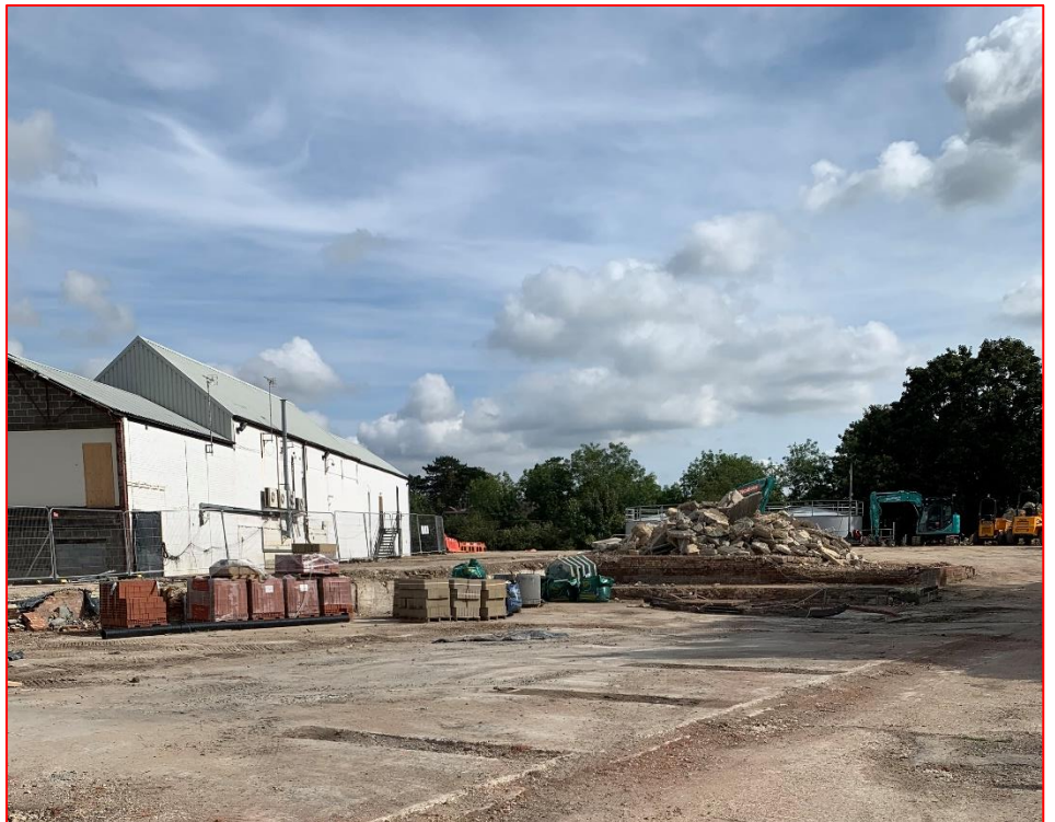
Plate 6 View of south elevation to the southernmost building within the application site (left). Note that this view is taken from Station Road looking east.
