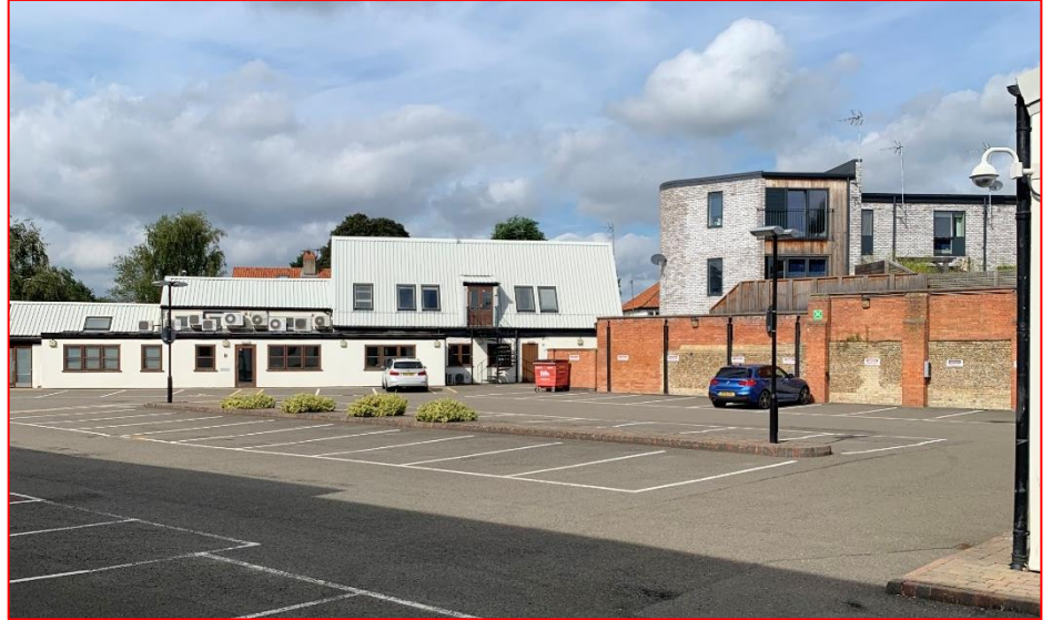
Plate 12 View looking west towards the east elevation of the westernmost building (centre-left) within the application site.
