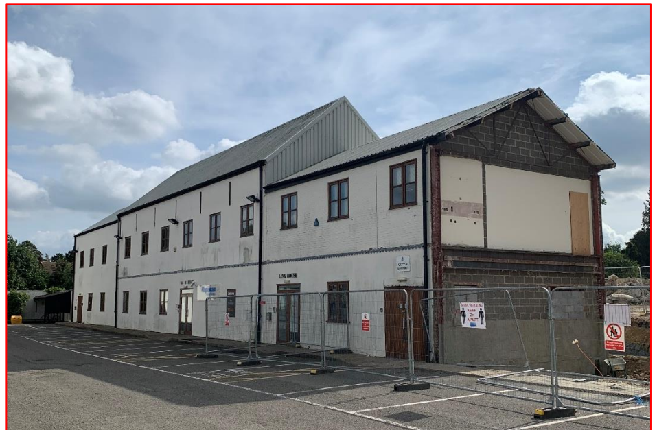
Plate 13 View of north elevation to the southernmost building within the application site. Note that this building has seen notable change over time.
