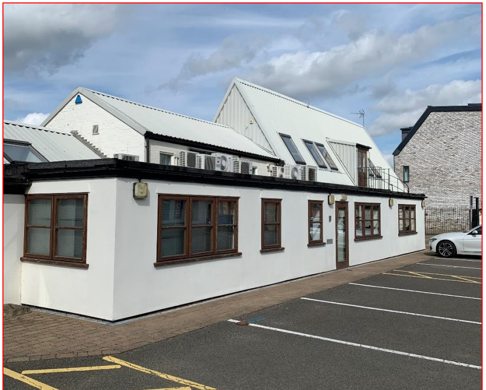
Plate 4 Existing east elevation to the westernmost building within the application site. Note that this view is taken from within the site looking north-west.
