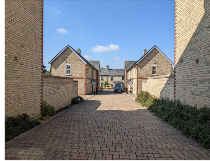
Fletcher's Way - Front Elevations within 8m of each other in a mews-type arrangement. Constructed 2014.
