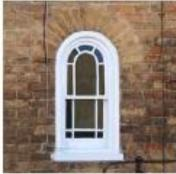
Later windows were of vertical emphasis, either divided into equal lights (left) or desented with narrow margin lights (sontrs). Lintels were often of gauged briekwork, Small, reunid-bauded windows (locally known as 'poor windows) are found on a number of bowes – wouldy tensords the from of a side wall
