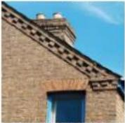
The eases of 19th convery houses were often deconsted. Higher startes beaux might have deep merhanging cases with wooden brackes (left). Simpler house had shallower cases with moddled bricks (convertey) or simple deg-tooth brickwork (contro becom). Gables might have simple deconstant (right).
