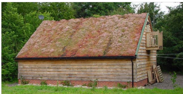
A private building using green roof techniques to lessen the visual impact.
