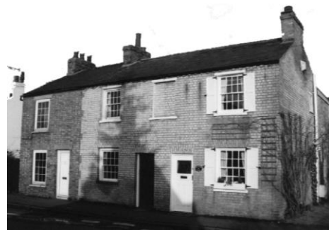
Nos. 1, 3 and 5 Station Road. No.1 has lost its original sash windows.
