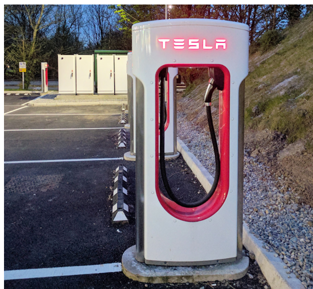
Fig. 26 | Electric vehicle charging point
