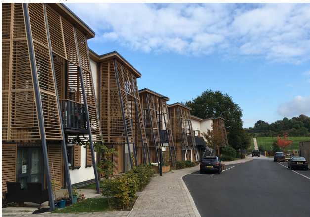
Fig. 51 | Exemplar sustainable buildings, Hanham Hall, Bristol
