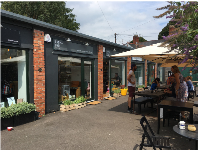
Fig. 54 | Retail units in light-weight, temporary structures with active outside spaces, Cardiff
