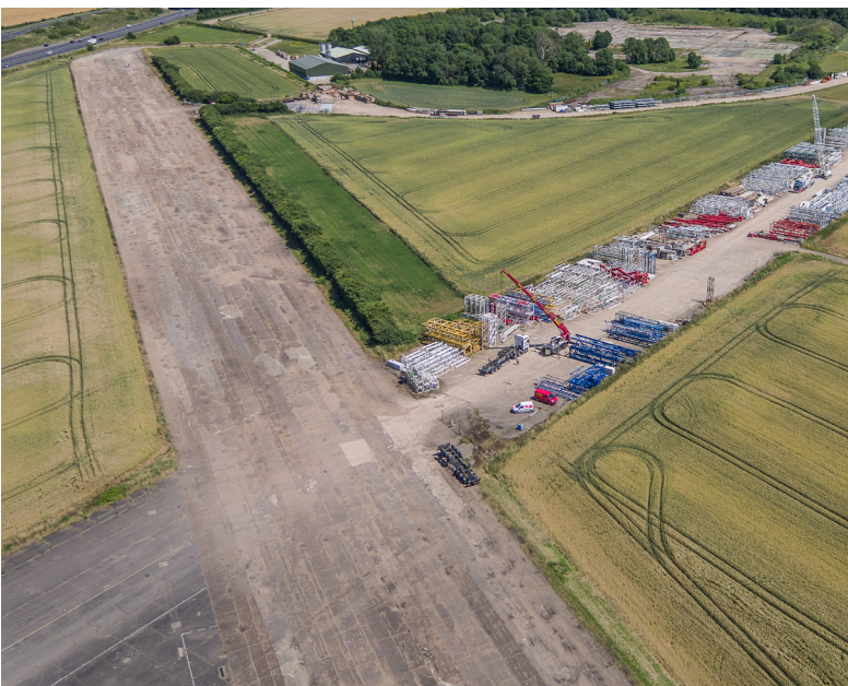
Fig. 41 | Overview of a section of the existing runway
