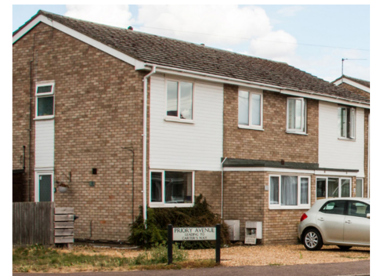
b. Priory Avenue: panels of white painted timber boarding are subservient to the full height brickwork, which turns the corner.
