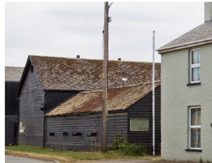
Figure 35: contrasts in the streetscape a. Boxworth End: agricultural buildings in continuous timber weatherboarding with black tar finish.
