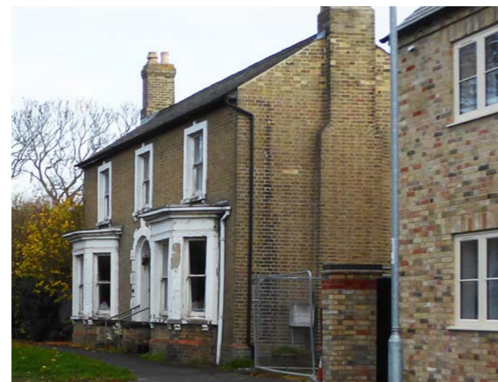
Figure 36: local accents a. Market Street: white render and paint to windows and projecting bays within a unified brick volume.
