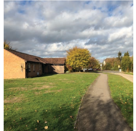
Figure 24. In Church Lane & Elm Way, typically single-storey dwellings face on to a series of pedestrian ways, car courts and passages. This is one version of a pedestrian focussed-design which appears throughout Papworth and which is accessible and pedestrian-friendly. New versions of this would be welcomed in new developments.
