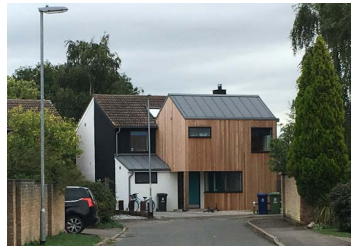
Figure 41 Recently constructed home in Over, an example of a complicated building envelope with multiple materials, not in keeping with village character.
